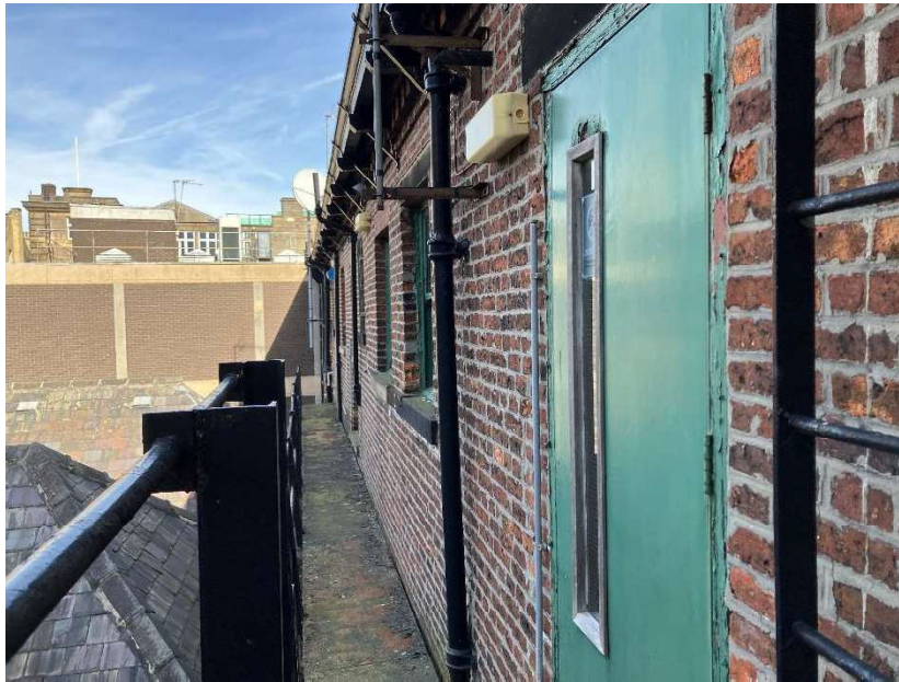
Image 1: View of first floor to rear of 2-14 New Street
