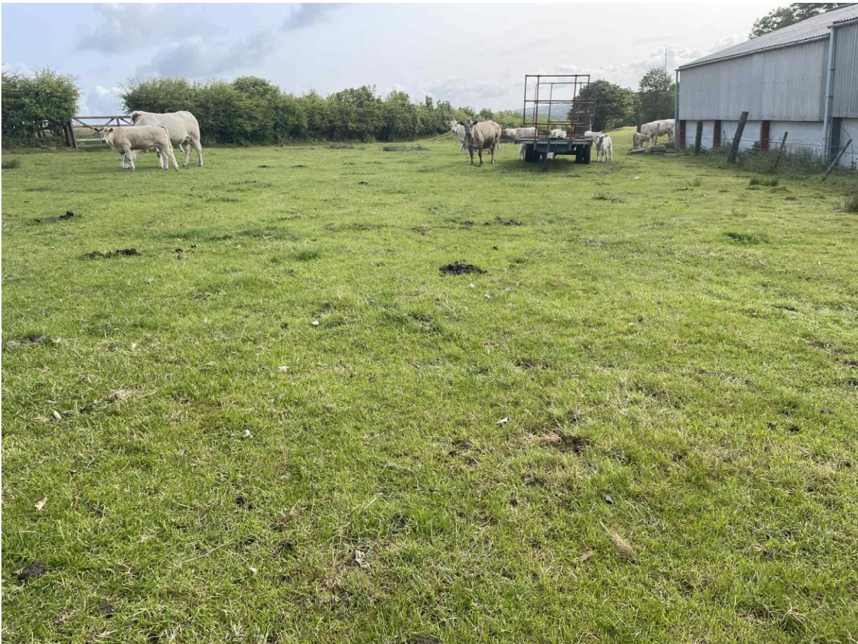
The proposed site from the west. The building is adjacent to the existing steep portal frame of similar proportions and constructed of the same materials.
