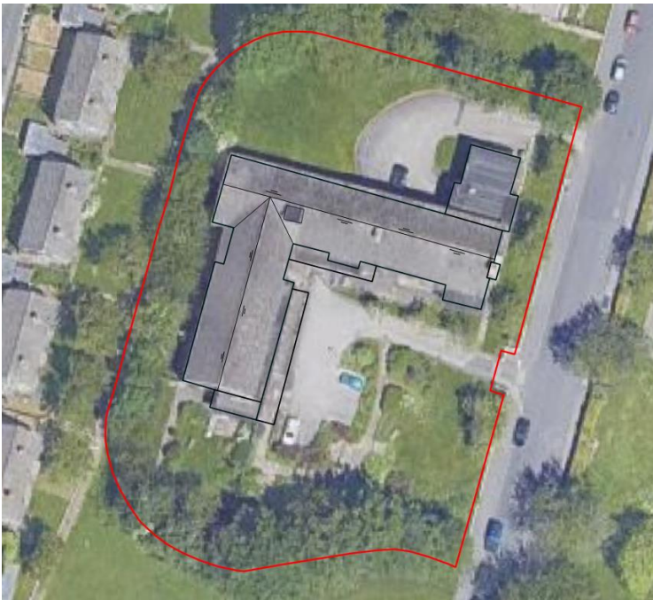
Figure 1 The surveyed building – red line
