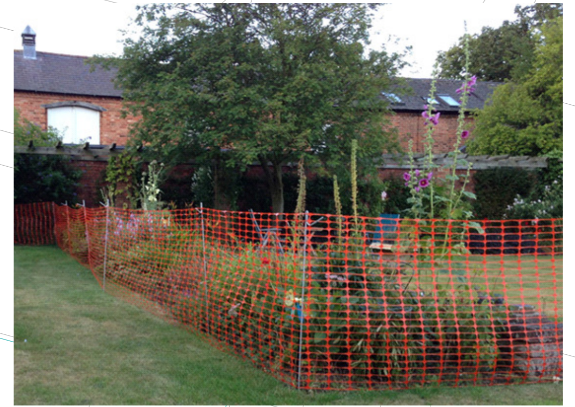
Inset 2: 'Mesh' Tree Protection Fencing
