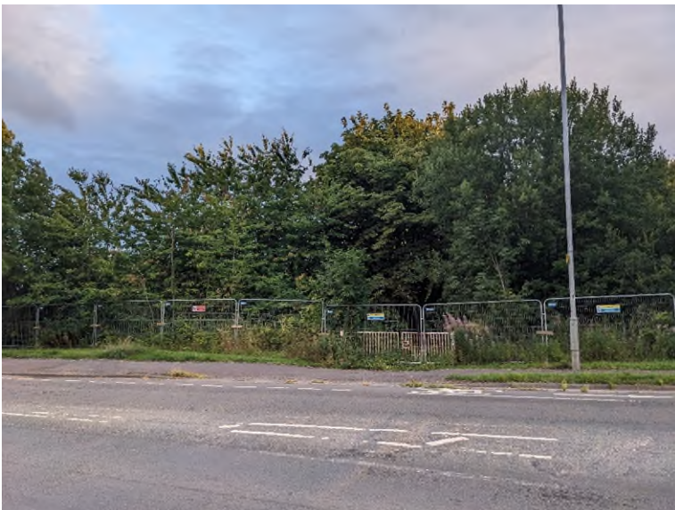
Photo 2 : Dropped Curb & Access Gate 2 Potential Access
