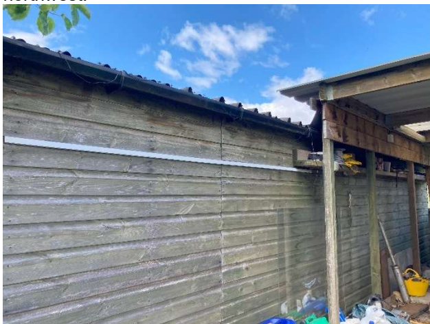
Photo 17: Building 4, viewed from the southeast.
