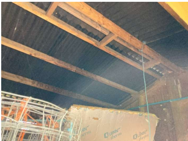
Photo 19: Interior of the western aspect of Building 4.
