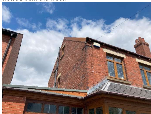
Photo 12: Building 1, viewed from the southwest.
