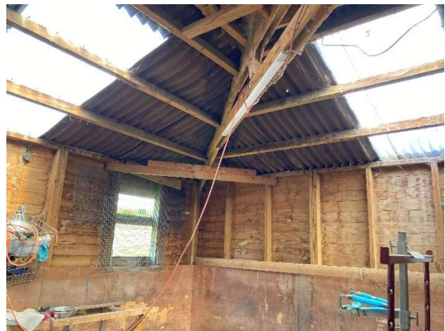
Photo 18: Interior of the northeastern aspect of Building 4.
