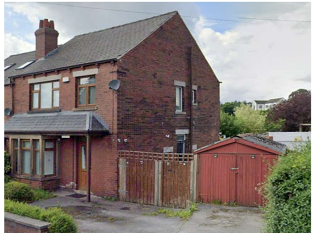
Photo 14: Building 2 and Building 3, viewed from the southeast.
