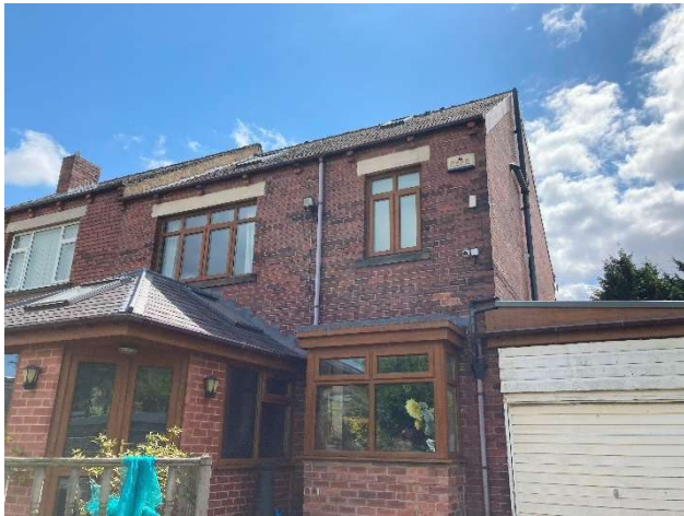
Photo 13: Building 1, viewed from the northwest.
