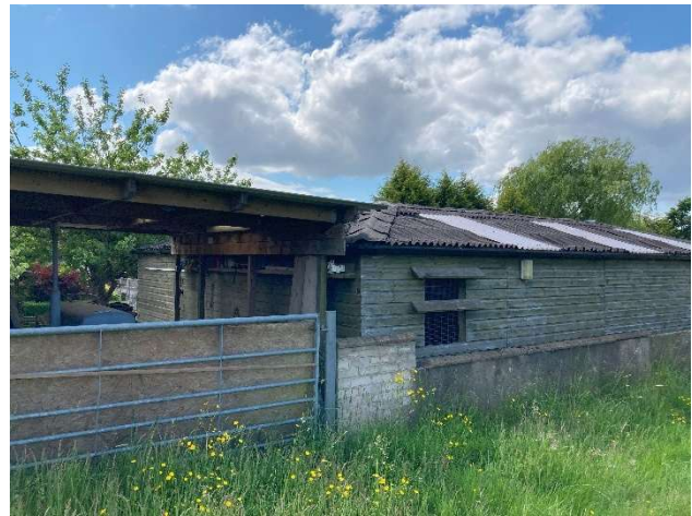
Photo 16: Building 4, viewed from the north.
