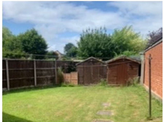
Photo 28: Building 5 & 6 viewed from the south.
