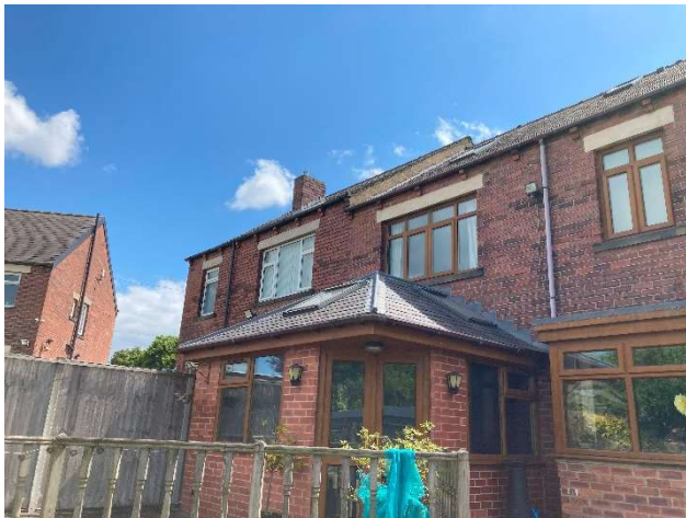
Photo 15: Building 1 and 2 viewed from the northwest.
