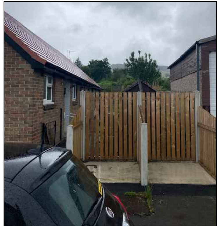
Photo showing the rear of no. 36 Olney Street and the new bin stores with the large garage adjacent the boundary line.
