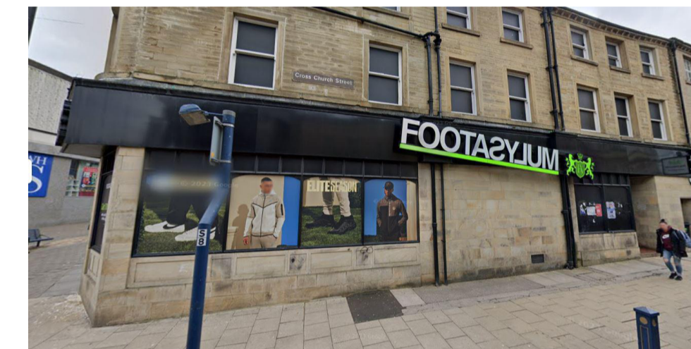
EXISTING SHOP FRONT - CROSS CHURCH STREET
