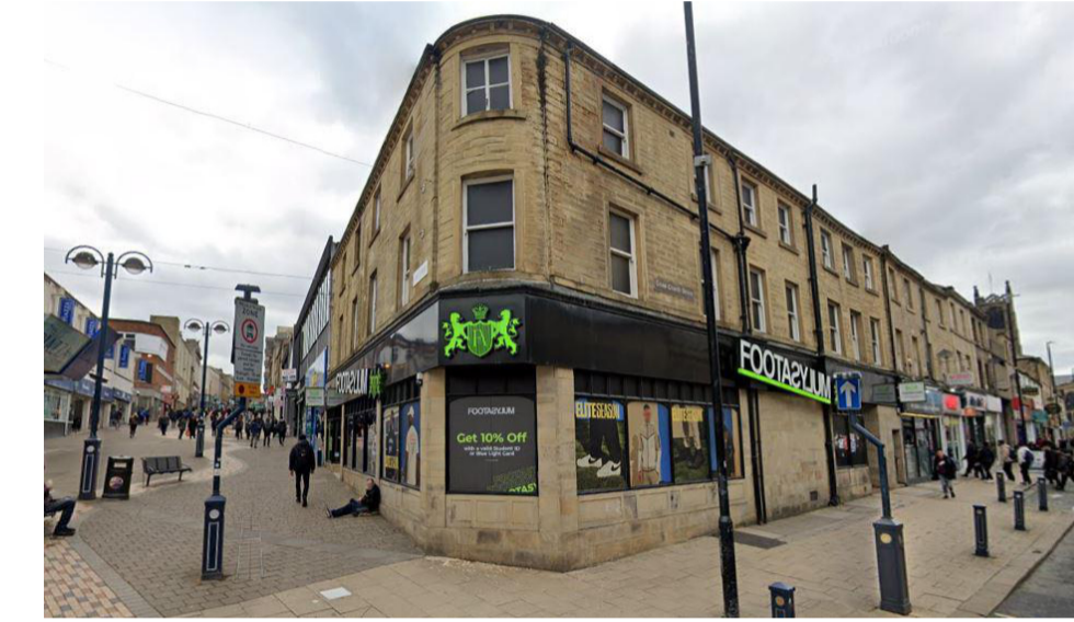
EXISTING SHOP FRONT - JUNCTION OF KING STREET & CROSS CHURCH STREET
