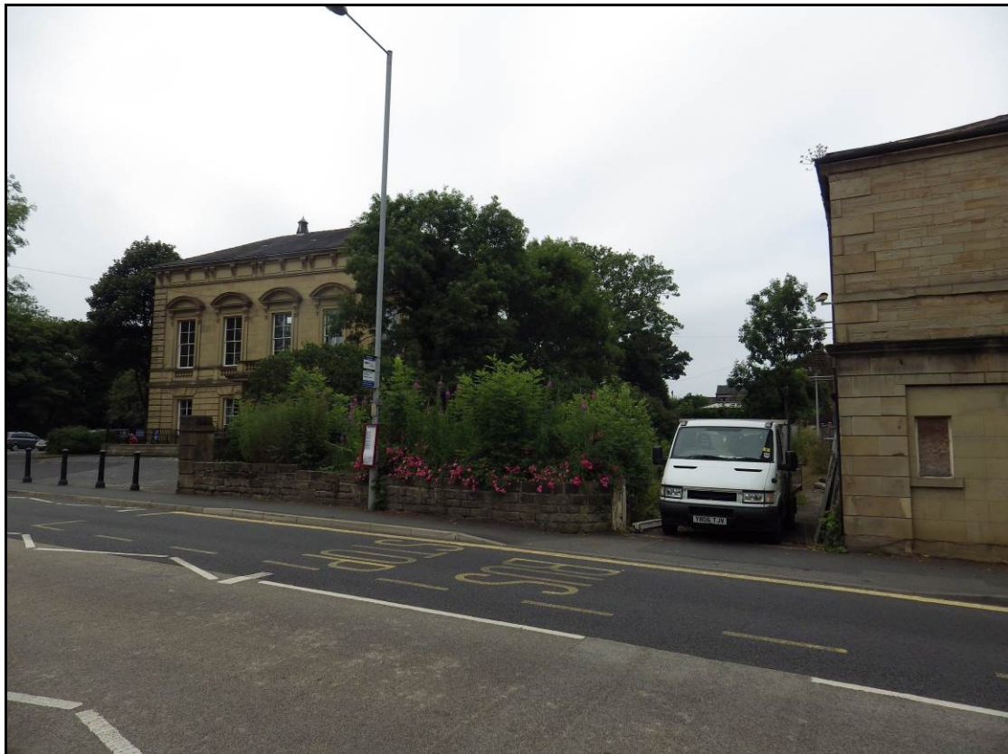
3.1.8. The photograph below looks from the overgrown lawn across the front of the site towards the school opposite.
