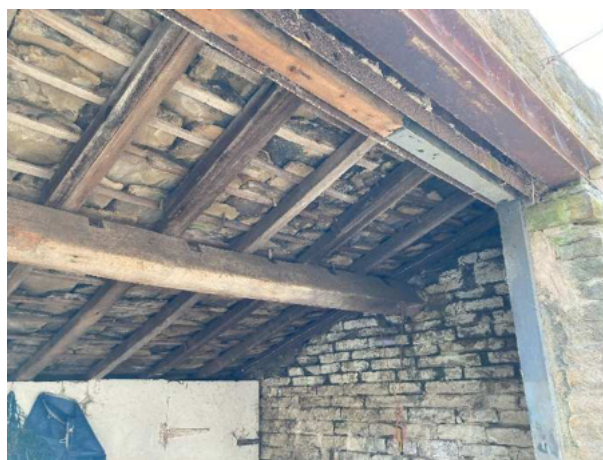
Photo 6: Interior of Building 2.
