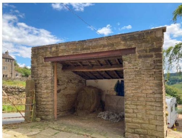
Photo 4: Building 2 and developed land sealed surface, viewed from the west.
