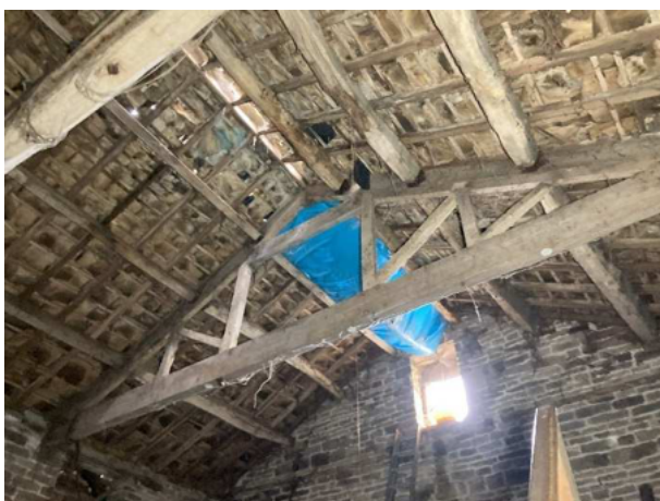
Photo 5: Interior of Building 1.
