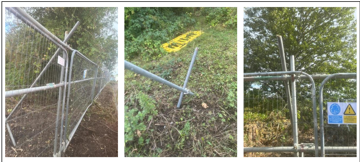
Figure A3.1: Examples of scaffold framework temporary tree protection fencing in-situ
