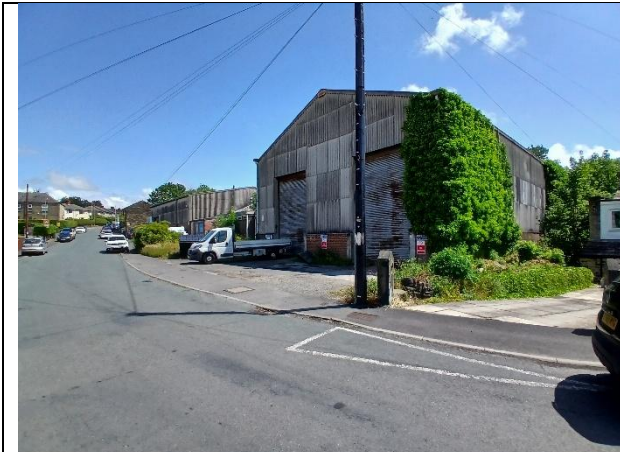
Photo 1: View of building 3 from the south.
