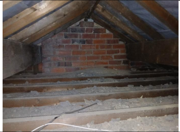
Photo 14: Inside the roof of building 1.
