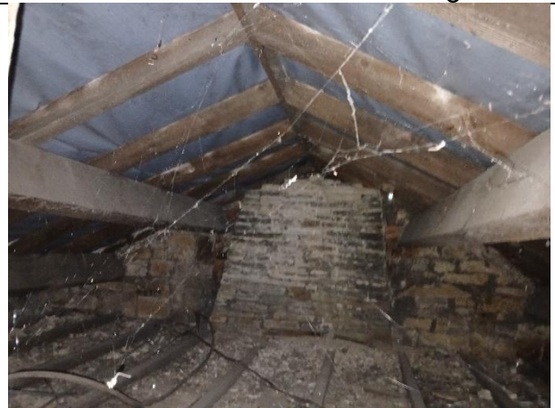
Photo 16: Inside the roof of building 1.
