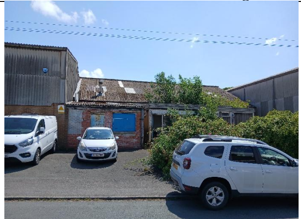
Photo 18: The extension of building 2.
