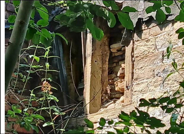
Photo 13: blocked up window of building 1.
