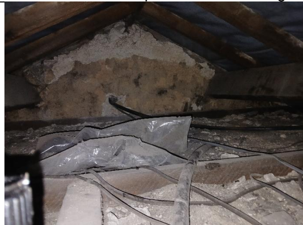
Photo 15: inside the roof of building 1.
