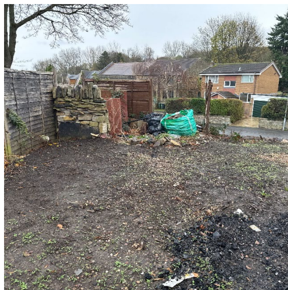
Figure 5: Photo showing the condition of the site in 2025.
