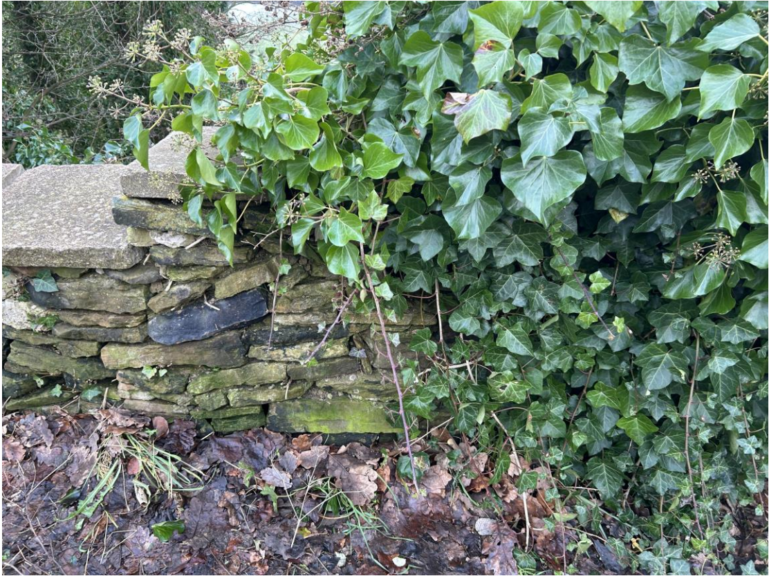
Photo 1 – Starting at Upper Section of Wall
