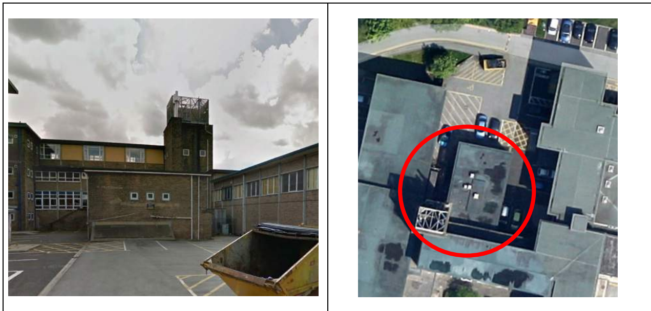
Figure 12: Former plant / boiler room location
