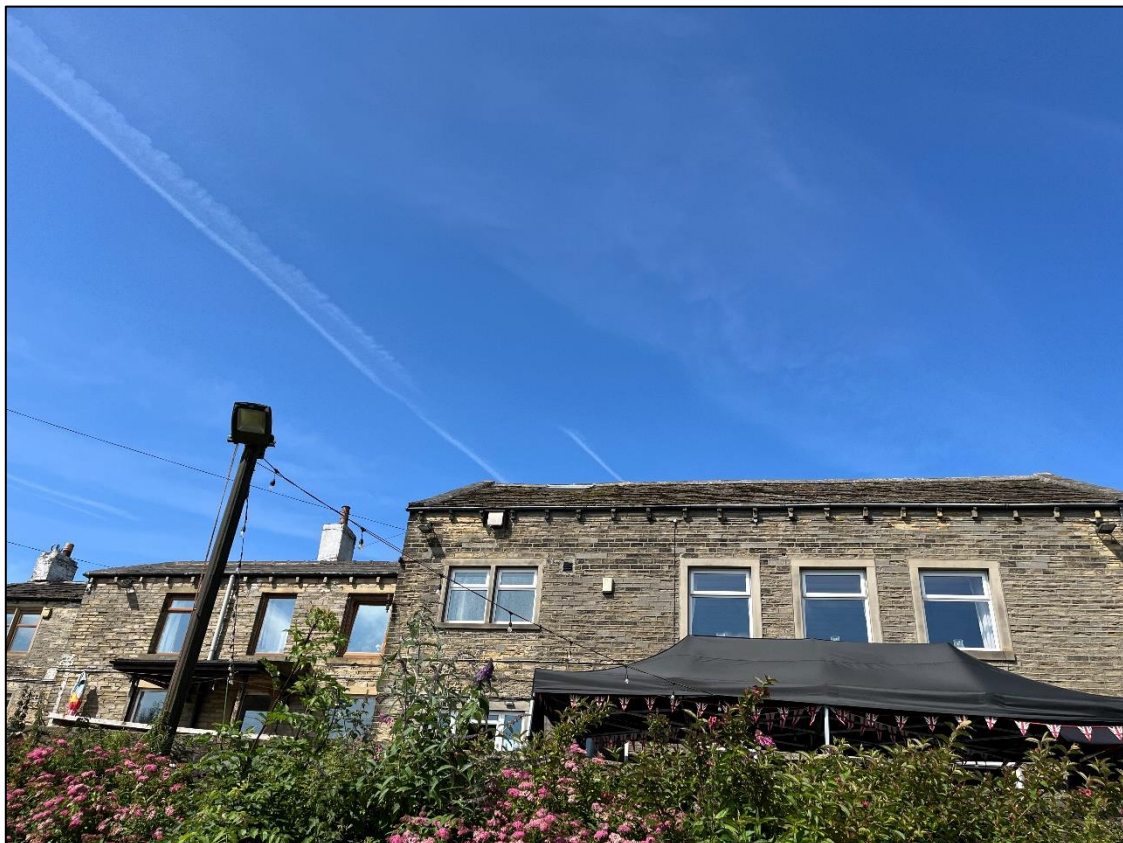
Plate 2 – Eastern aspect of the building
