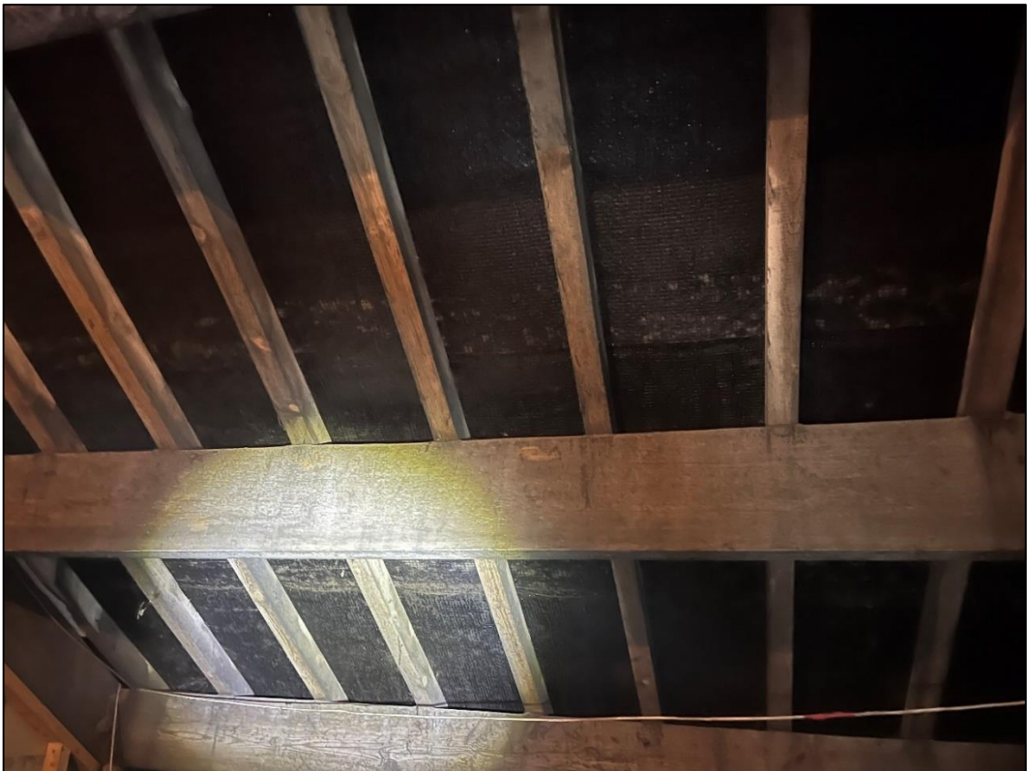
Plate 6 – Bitumen lining within loft spaces
