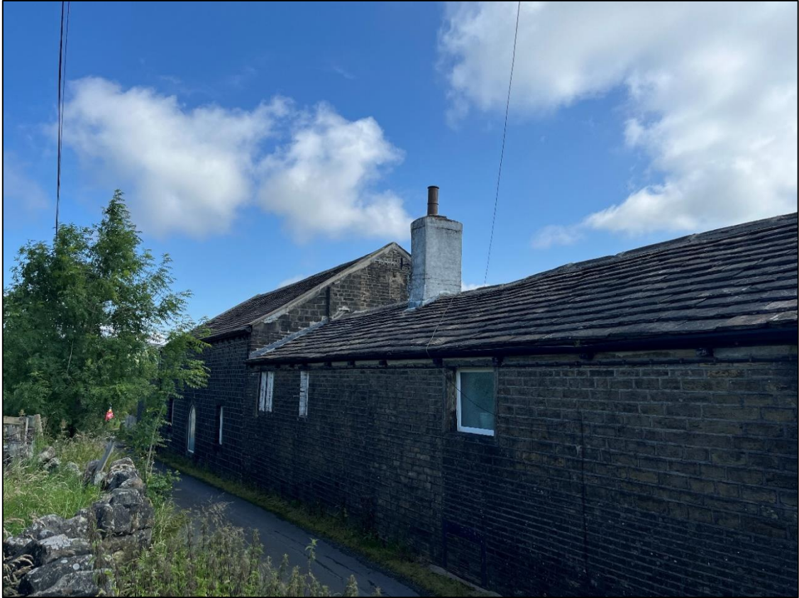
Plate 3 – Western elevation of the building
