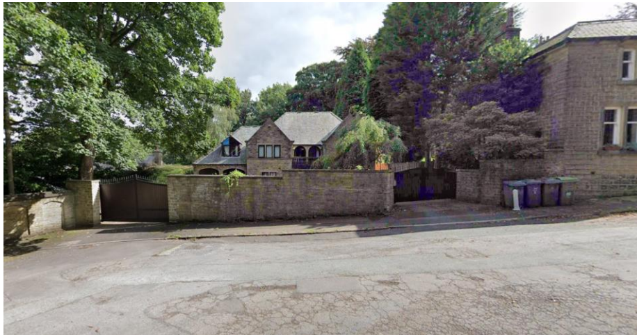
Existing Stone Wall Screen of 2 Kaffir Road, Taken From the 90 Degree Corner, Google Maps
