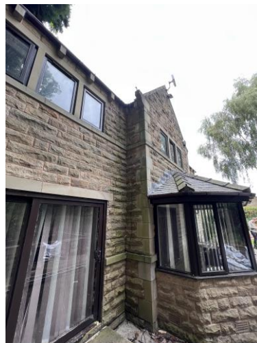
Stone Heads, Cills, Mullions and Quoins Shown on Front and Rear External Walls
