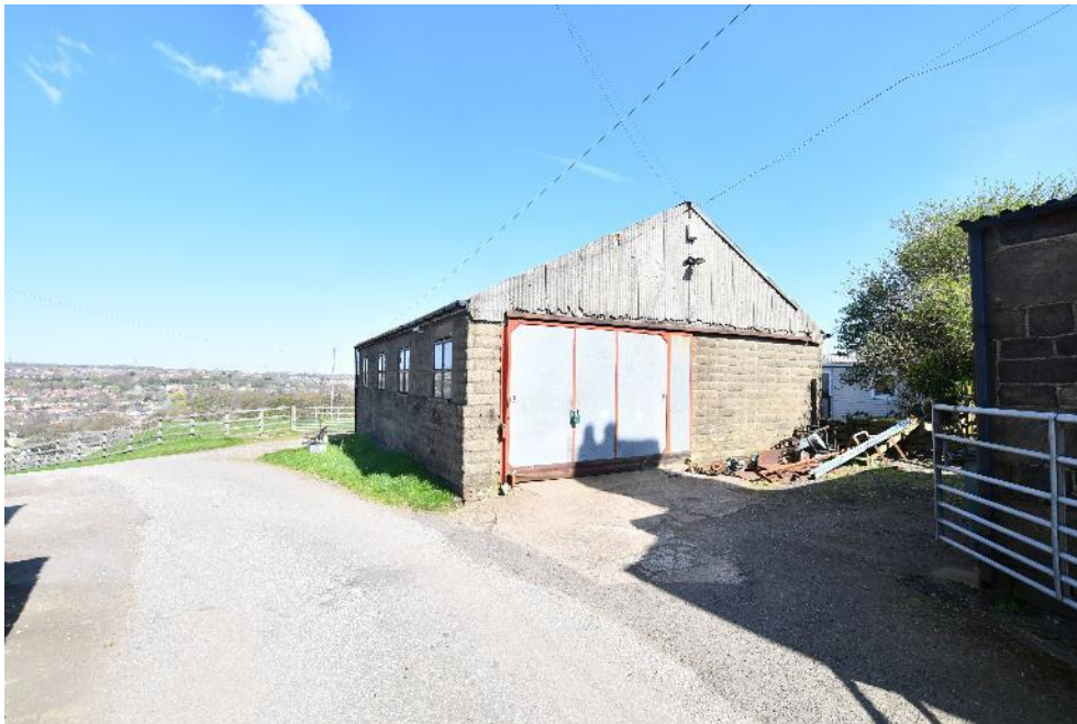
Image 4 Small Workshop with skylights and windows
