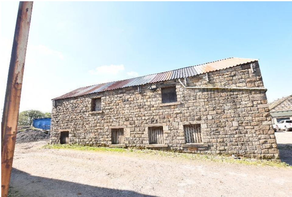
Image 6 Large Stone built barn with metal roof – to be retained
