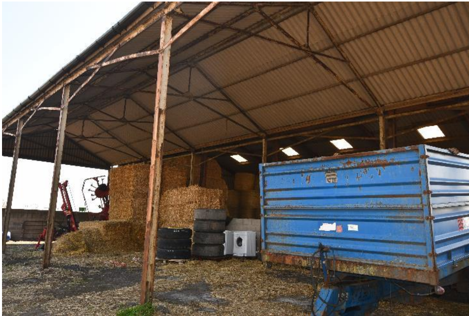
Image 1 Large open fronted barn with corrugated roof and skylights in rear section
