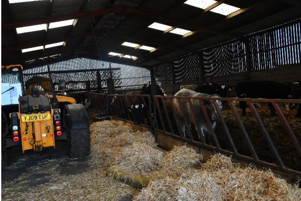
Image 5 Internal structure of large barn with Yorkshire Boarding Skylights and corrugated roof
