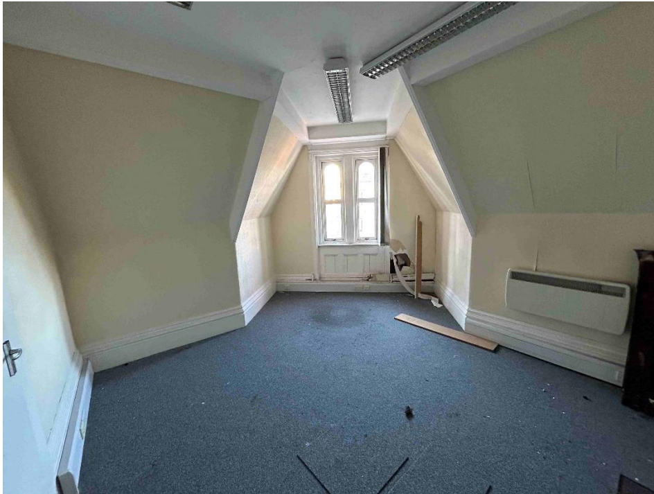
PHOTOGRAPH 18 – Modern fixtures To be removed. Window Surrounds and Panelling to Remain. Skirtings to be restored / replaced.
