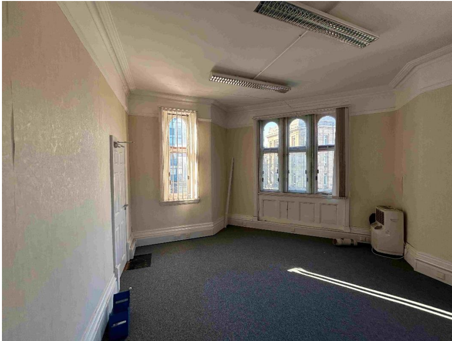
PHOTOGRAPH 9 – Modern fixtures To be removed. Window Surrounds and Panelling to Remain. Skirtings to be restored / replaced. Cornice and Picture Rail to Remain.
