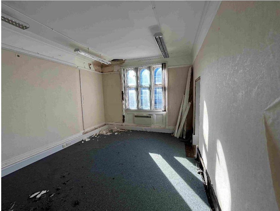
PHOTOGRAPH 11 – Modern fixtures To be removed. Window Surrounds and Panelling to Remain. Skirtings to be restored / replaced. Cornice and Picture Rail to Remain. Chimney Breast to Remain
