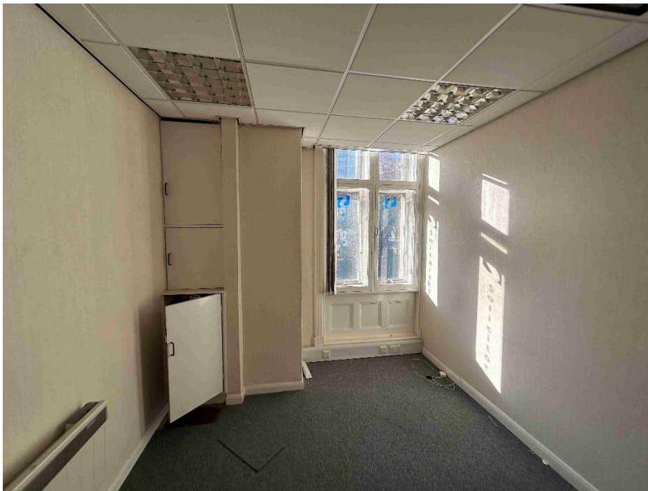
PHOTOGRAPH 4 – Modern fixtures and partitions to be removed. Window Surrounds and Panelling to Remain. Skirtings to be replaced.
