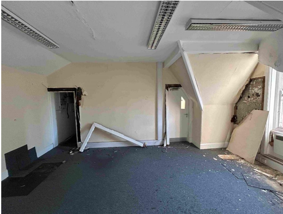
PHOTOGRAPH 20 – Modern fixtures To be removed. Window and Door Surrounds and Panelling to Remain. Skirtings to be restored / replaced. Chimney Breast to Remain. Roof to be repaired.
