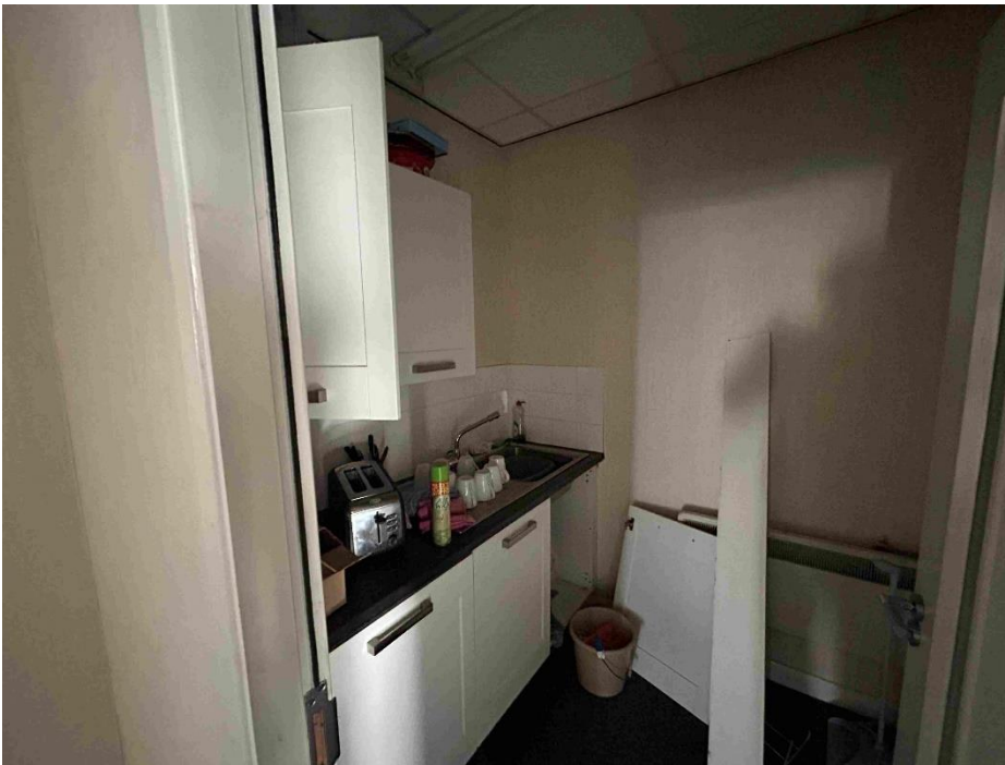
PHOTOGRAPH 6 – Modern fixtures and partitions to be removed.
