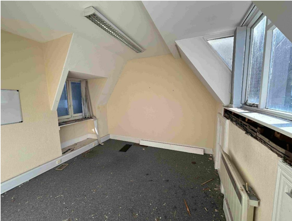
PHOTOGRAPH 22 – Modern fixtures To be removed. Window Surrounds Remain.
