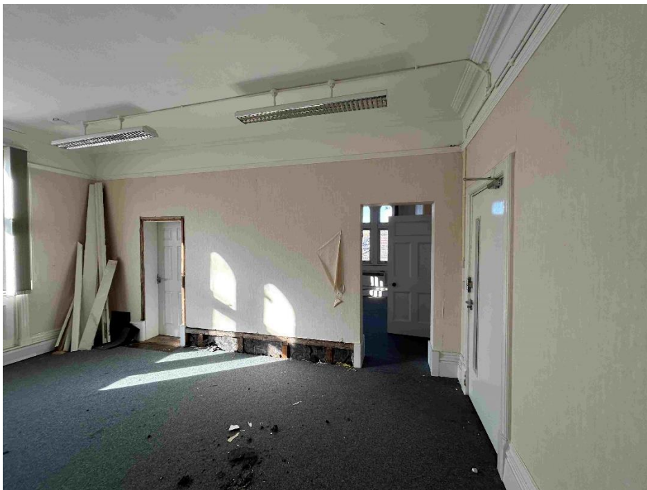
PHOTOGRAPH 12 – Modern fixtures To be removed. Window Surrounds and Panelling to Remain. Skirtings to be restored / replaced. Cornice and Picture Rail to Remain.
