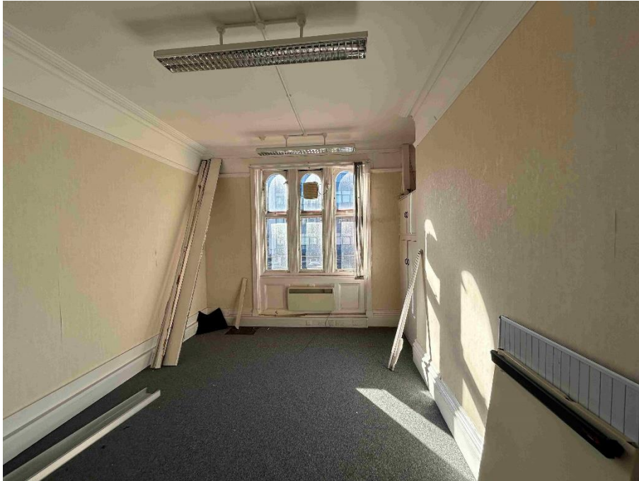
PHOTOGRAPH 13 – Modern fixtures To be removed. Window Surrounds and Panelling to Remain. Skirtings to be restored / replaced. Cornice and Picture Rail to Remain. Chimney Breast to Remain.
