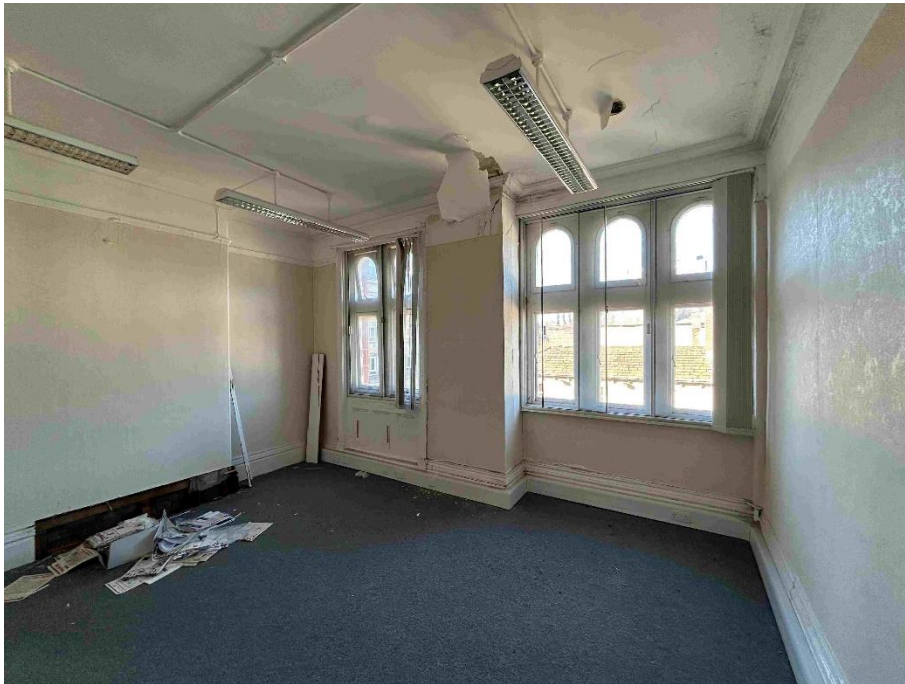
PHOTOGRAPH 7 – Modern fixtures To be removed. Window Surrounds and Panelling to Remain. Skirtings to be restored / replaced. Cornice and Picture Rail to Remain. Chimney Breast to Remain
