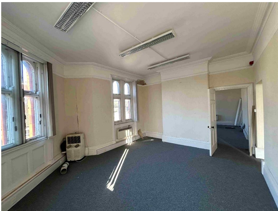
PHOTOGRAPH 10 – Modern fixtures To be removed. Door and Window Surrounds and Panelling to Remain. Skirtings to be restored / replaced. Cornice and Picture Rail to Remain. Chimney Breast to Remain
