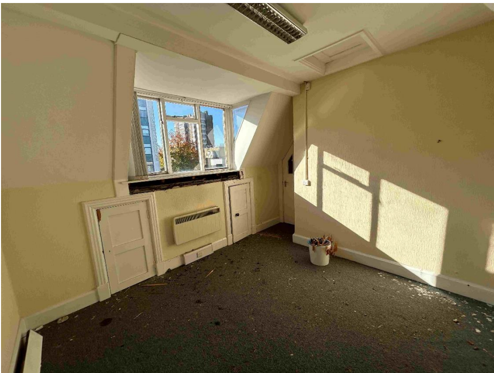
PHOTOGRAPH 23 – Modern fixtures To be removed. Window and Door Surrounds Remain
