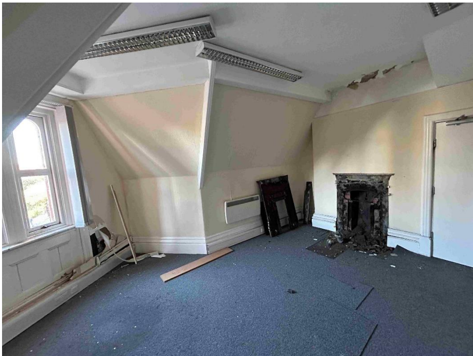
PHOTOGRAPH 19 – Modern fixtures To be removed. Window and Door Surrounds and Panelling to Remain. Skirtings to be restored / replaced. Chimney Breast to Remain
