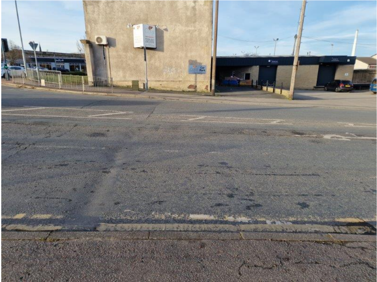
Lower Fitzwilliam Street/ Southgate junction (west side at the lights)
