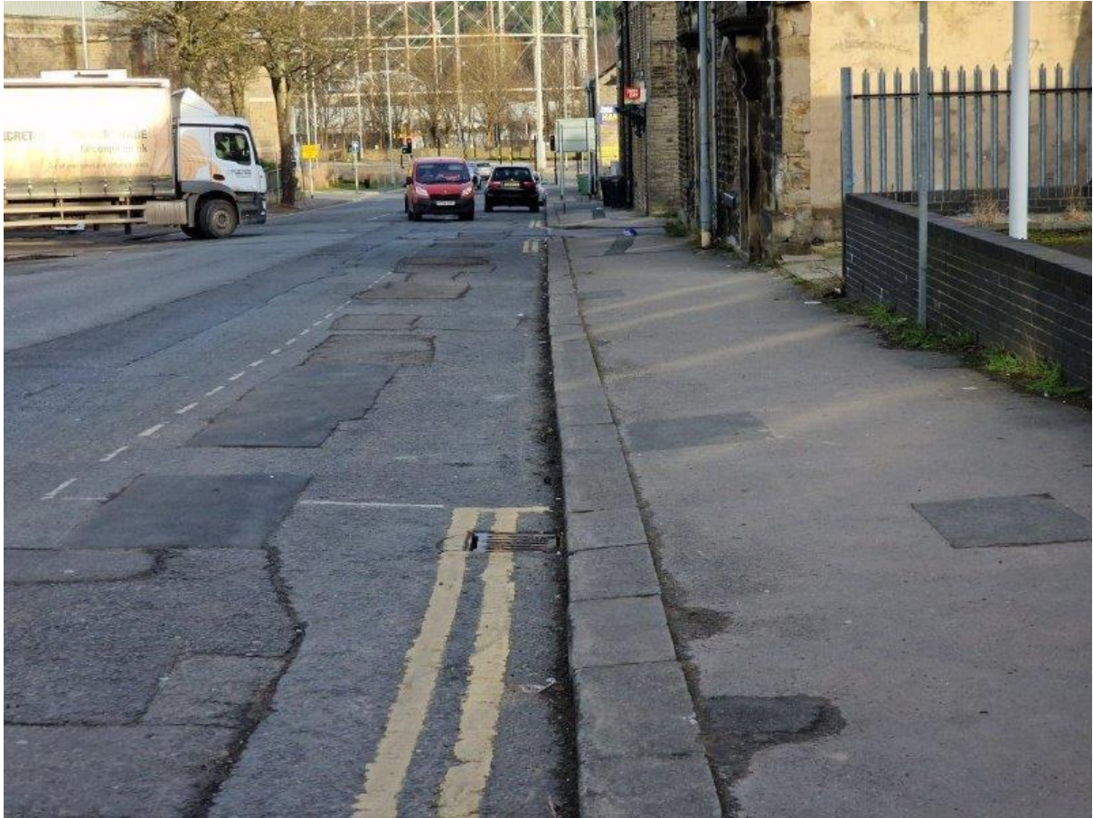
Lower Fitzwilliam Street/William Street junction south east side
