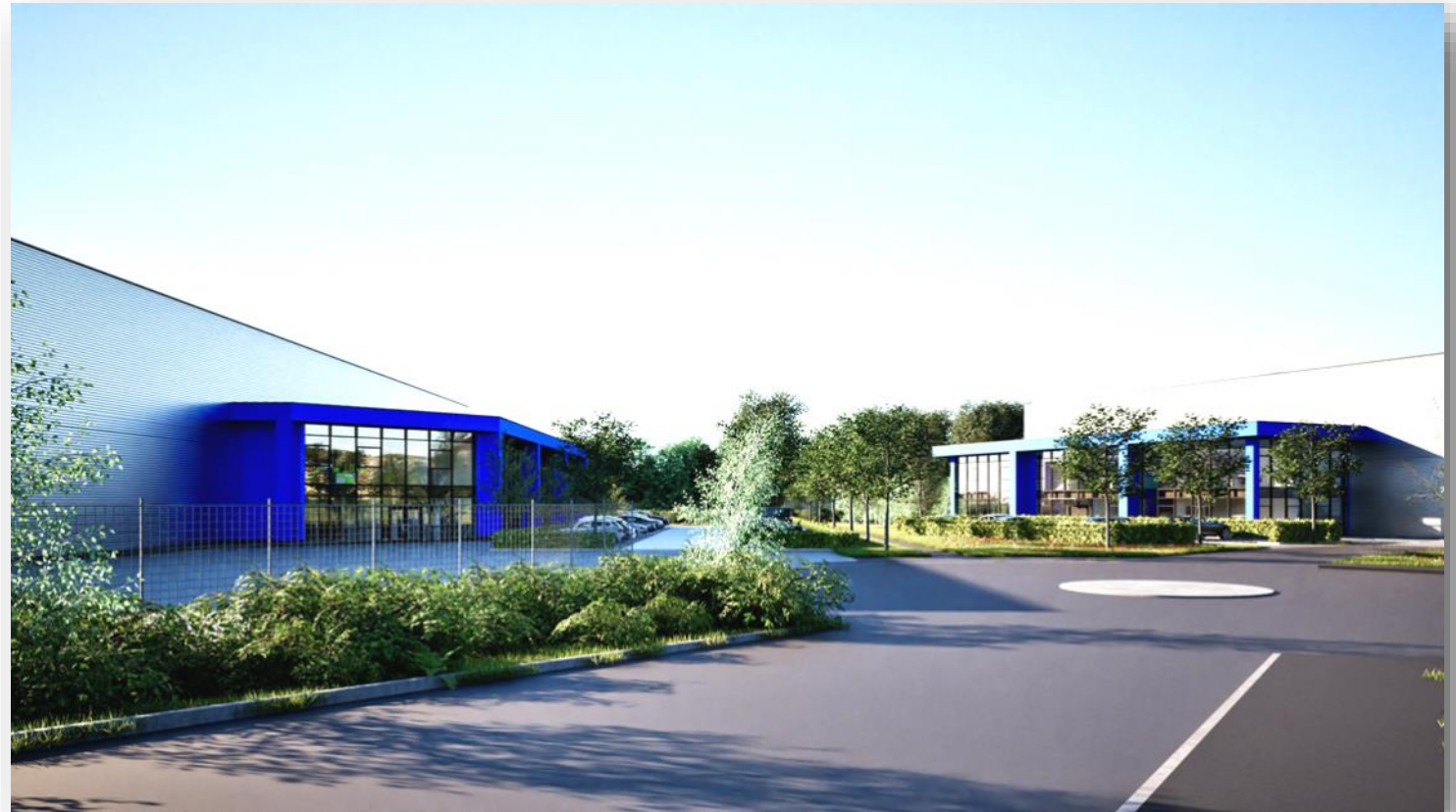
View from access road
