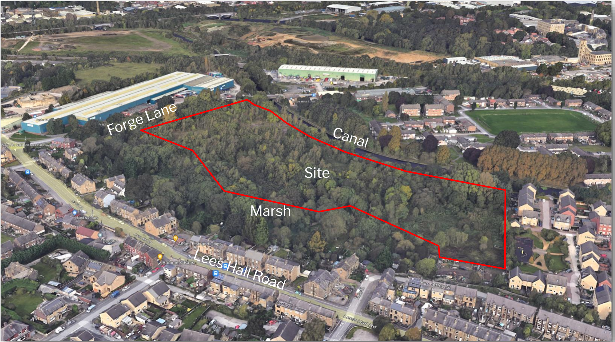
View from the South
