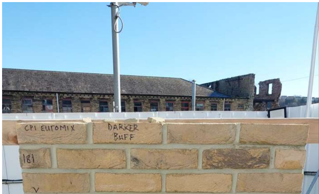
Fig. 3) Plant room brick and mortar sample
