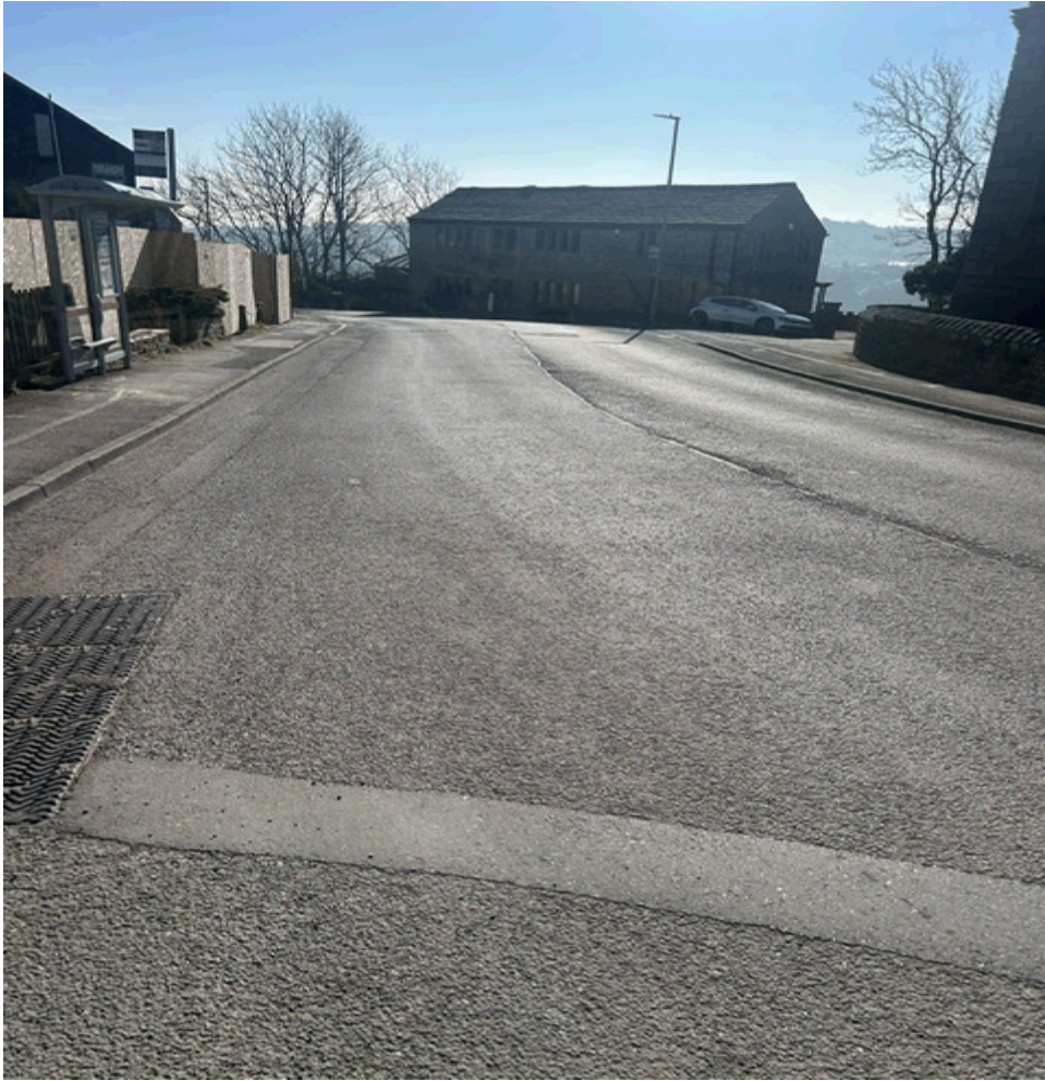
ROADWAY LOOKING EAST TO KNOWL ROAD
