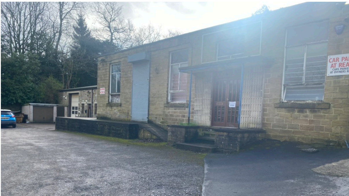
Photo 2 – View toward existing engineering works
