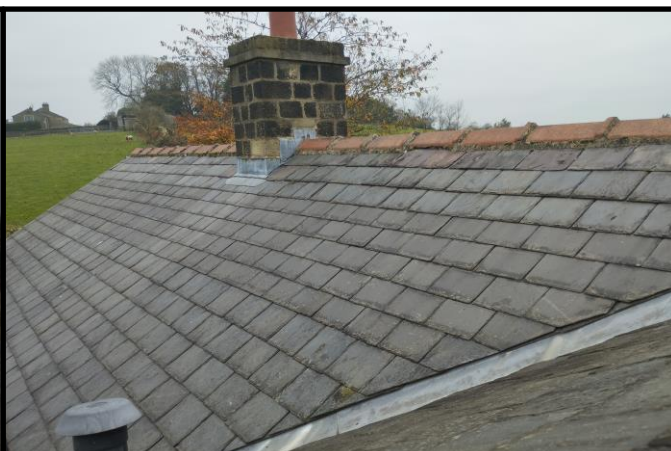
Photograph 2. Example of roof
