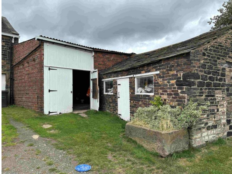
Photograph 1 – View From the South
