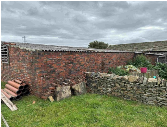
Photograph 5 – View of North West Corner
