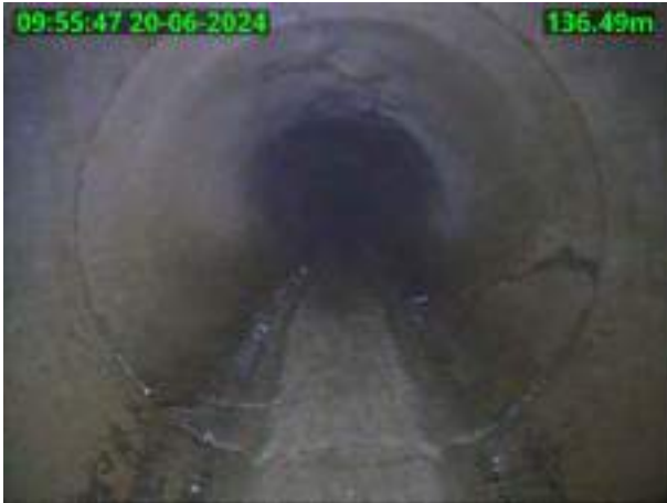
(CL) Crack longitudinal at ... o'clock ./.MH101-Pipe---X/MH101-Pipe---X_2024_06_20- (MH) Manhole/node ./.MH101-Pipe---X/MH101-Pipe---X_2024_06_20-
