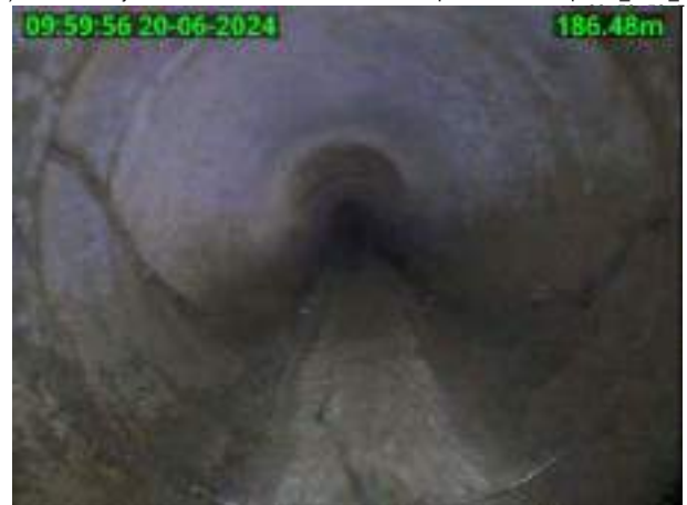
(CL) Crack longitudinal at ... o'clock ./.MH101-Pipe---X/MH101-Pipe---X_2024_06_20- (MH) Manhole/node ./.MH101-Pipe---X/MH101-Pipe---X_2024_06_20-
