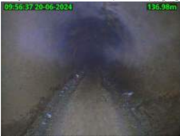
(RFJ) Roots fine at joint ./.MH101-Pipe---X/MH101-Pipe---X_2024_06_20- (RFJ) Roots fine at joint ./.MH101-Pipe---X/MH101-Pipe---X_2024_06_20-
