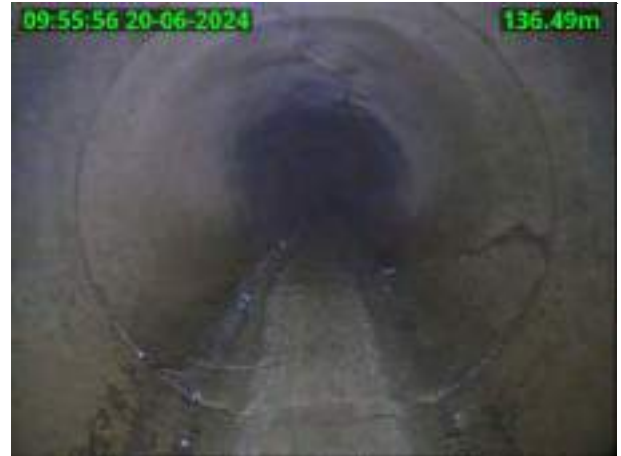
(CL) Crack longitudinal at ... o'clock ./.MH101-Pipe---X/MH101-Pipe---X_2024_06_20- (MH) Manhole/node ./.MH101-Pipe---X/MH101-Pipe---X_2024_06_20-
