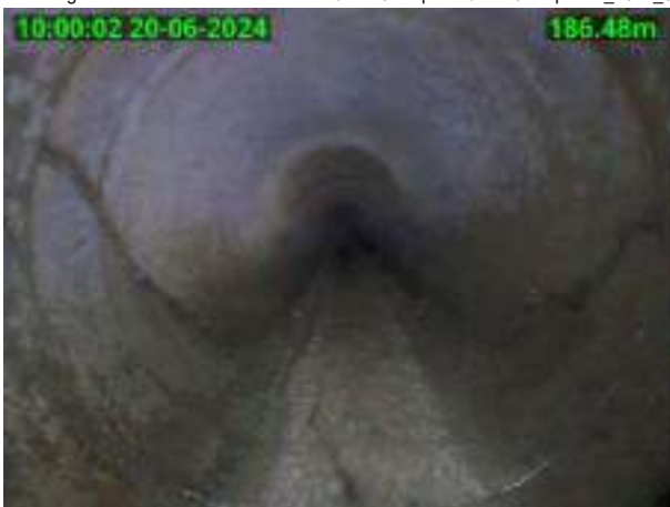
(CL) Crack longitudinal at ... o'clock ./.MH101-Pipe---X/MH101-Pipe---X_2024_06_20- (MH) Manhole/node ./.MH101-Pipe---X/MH101-Pipe---X_2024_06_20-
