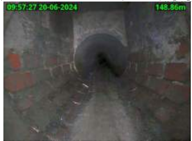
(RFJ) Roots fine at joint ./.MH101-Pipe---X/MH101-Pipe---X_2024_06_20- (RFJ) Roots fine at joint ./.MH101-Pipe---X/MH101-Pipe---X_2024_06_20-
