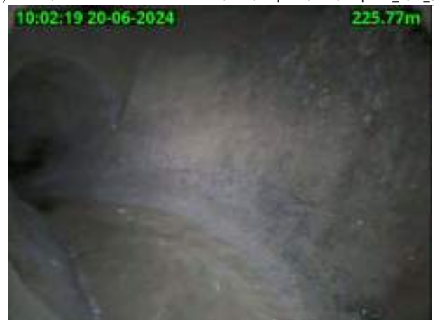
(CL) Crack longitudinal at ... o'clock ./.MH101-Pipe---X/MH101-Pipe---X_2024_06_20- (MH) Manhole/node ./.MH101-Pipe---X/MH101-Pipe---X_2024_06_20-
