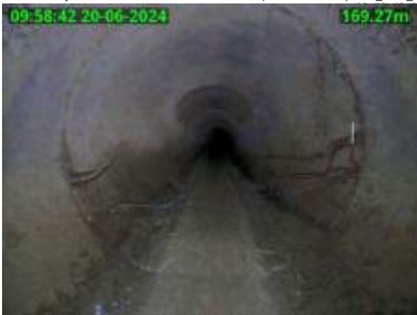
(CL) Crack longitudinal at ... o'clock ./.MH101-Pipe---X/MH101-Pipe---X_2024_06_20- (MH) Manhole/node ./.MH101-Pipe---X/MH101-Pipe---X_2024_06_20-
