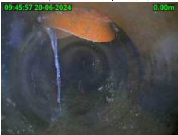
(H) Hole in sewer at ... (OR from ... to ...) ./.MH101-Pipe---X/MH101-Pipe---X_2024_06_20- (CL) Crack longitudinal at ... o'clock ./.MH101-Pipe---X/MH101-Pipe---X_2024_06_20-
