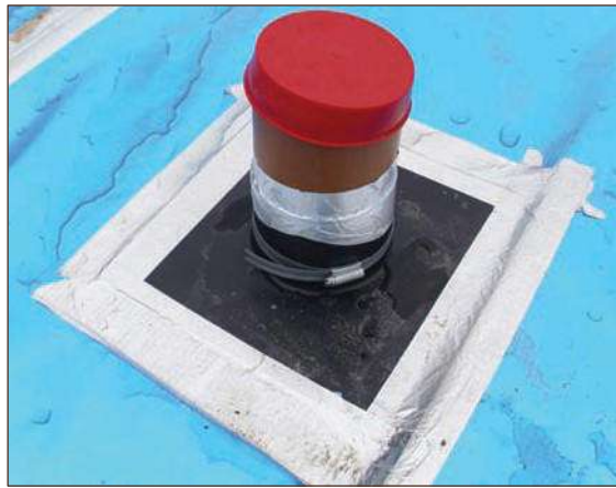
Figure A4.26 Well-constructed service entry: top hat fits well with service pipe and taped down to gas membrane, secondary seal with proprietary single sided tape (courtesy Smith Grant)
