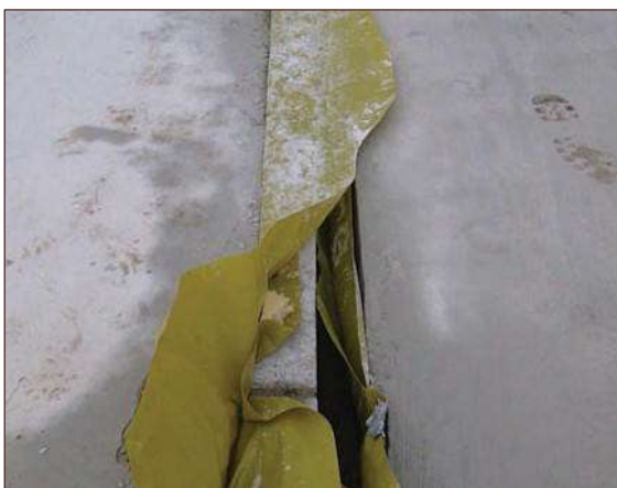
Figure A4.79 Gas membrane not continuous over internal wall. It had been deliberately cut open for unknown purpose (courtesy Smith Grant)
