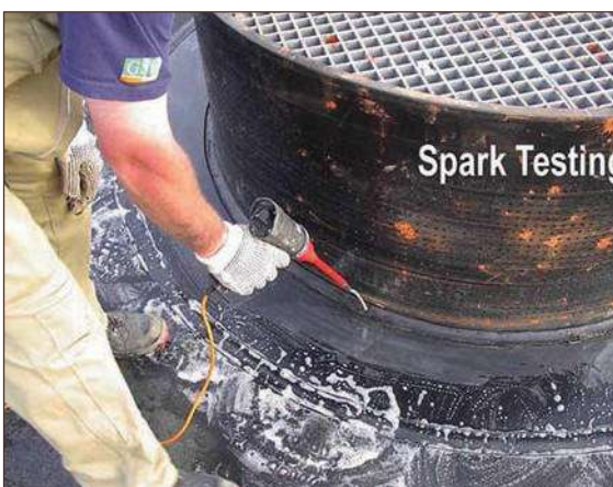
Figure A4.45 Spark testing (courtesy GSE Environmental)
