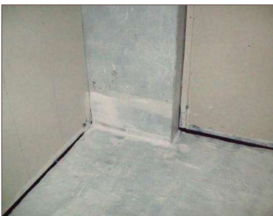
Figure A4.83 Poor quality installation of liquid gas membrane. Liquid gas membranes come in two colours (black and white) allowing coverage of each coat to be easily assessed. Here the gas membrane has been spread too thinly and inconsistently. In addition, it appears to have been applied to a damp surface, causing blistering (courtesy Card Geotechnics Limited)
