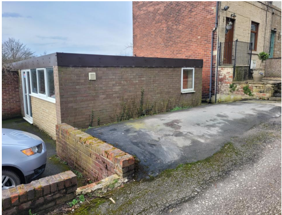
Front elevation of existing building
