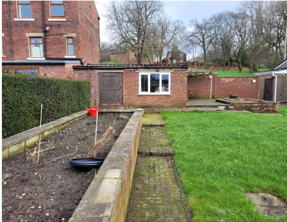
Rear elevation of existing building
