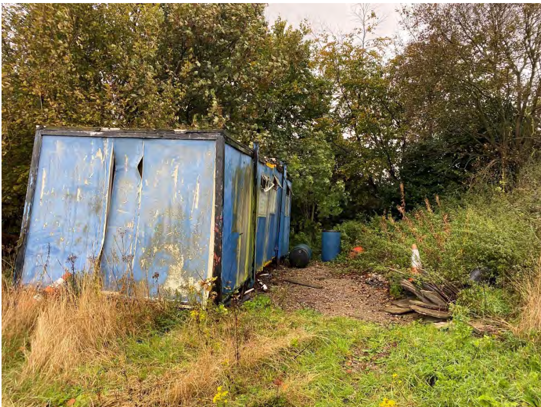
Photo 8. Looking north-west towards container and trees in north-eastern corner of site
