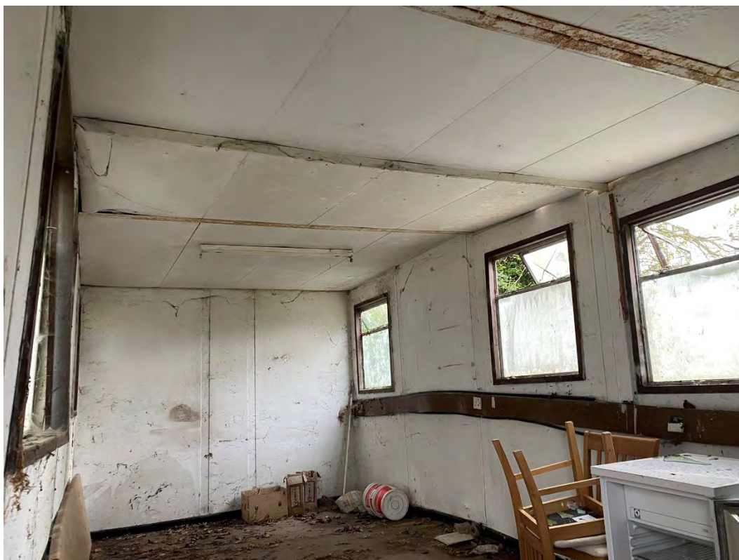
Photo 12. Interior of the container in north-east corner of the site
