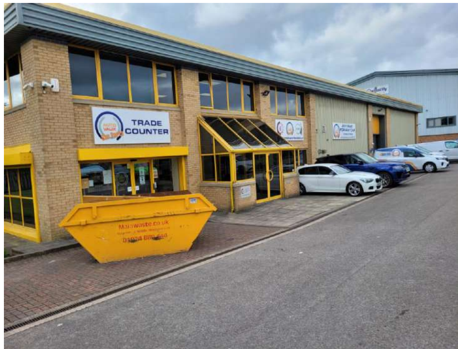
View of front of building looking to the south
