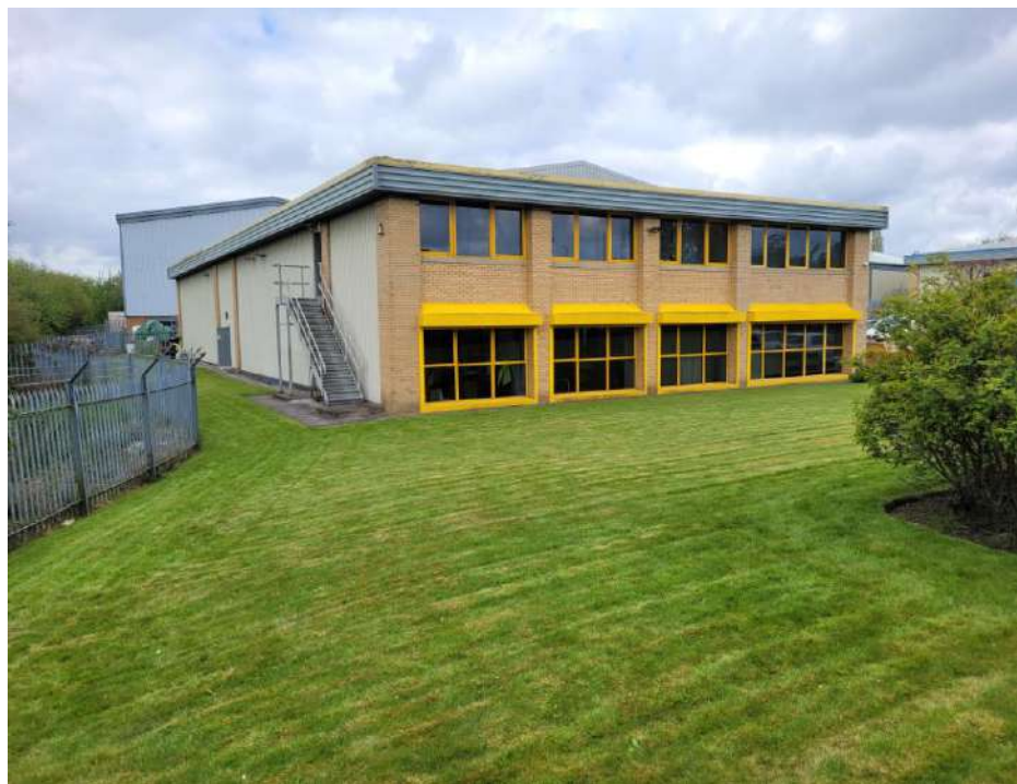
Area adjacent to northeastern boundary
