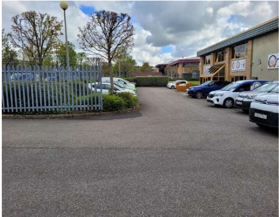
View of front of building looking to the east
