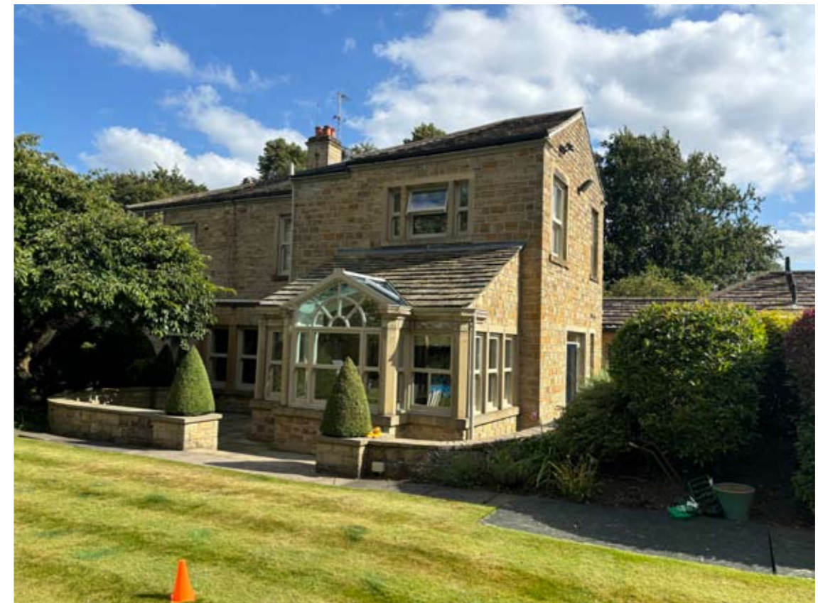
Figure 4 – North view of 289 Oxford Road
