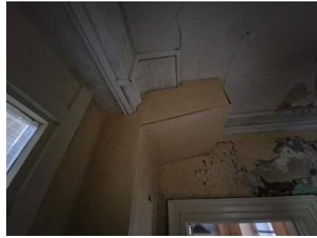
Partition wall beneath stairs to separate corridor and bulkhead detail to cover stairs as part of the children's care home development
