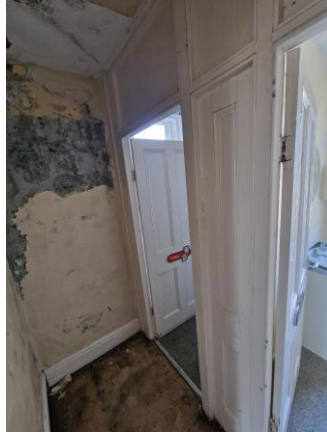
WC and bathroom partition
