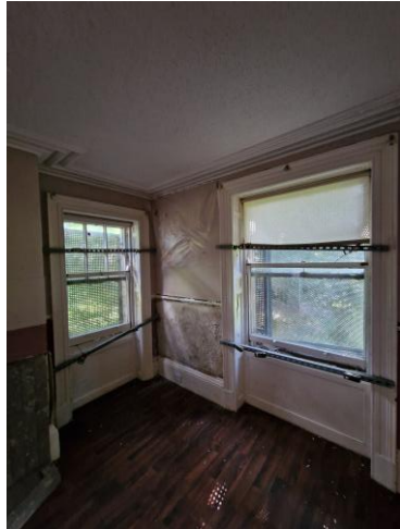
Sash windows with the window (left) having six sections on the upper pane
