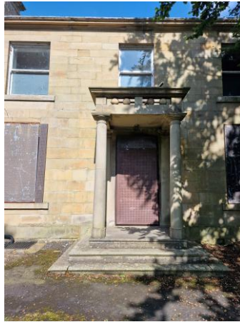
Tuscan porch over front entry
