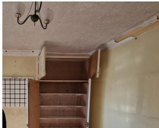
Timber coping on the right side of the image seen with paint stripping away
