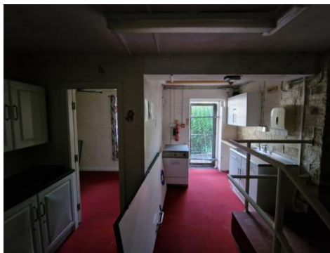
Existing utility room in old garage
