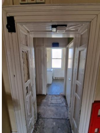
Opening between buildings 1 and 2a/2b
