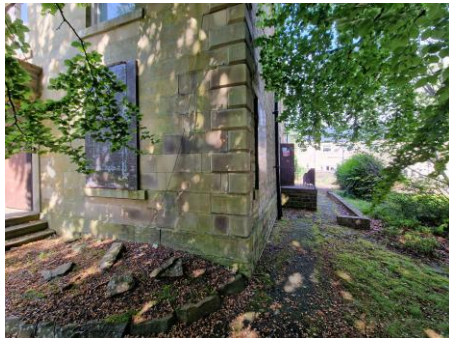
Quoins on the south-east corner facade
