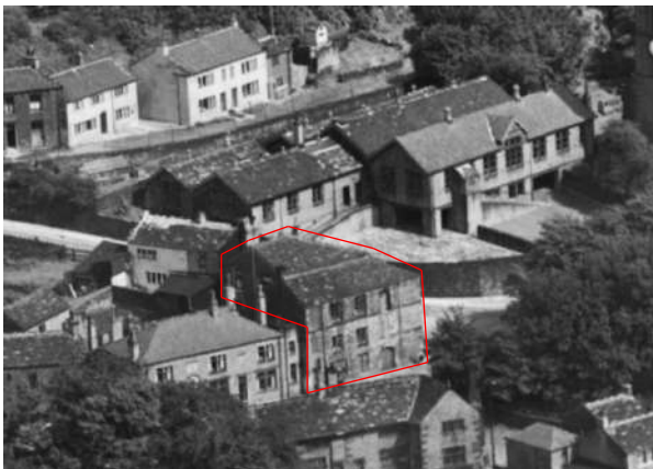
Figure 6: Britain from Above - EAW018228 ENGLAND (1948). Upper Mill and environs, Slaithwaite, 1948.
