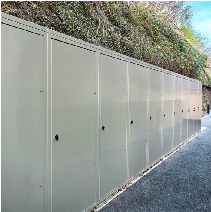
Photograph 4 – Example of Secure Cycle Storage in Basement Parking Area
