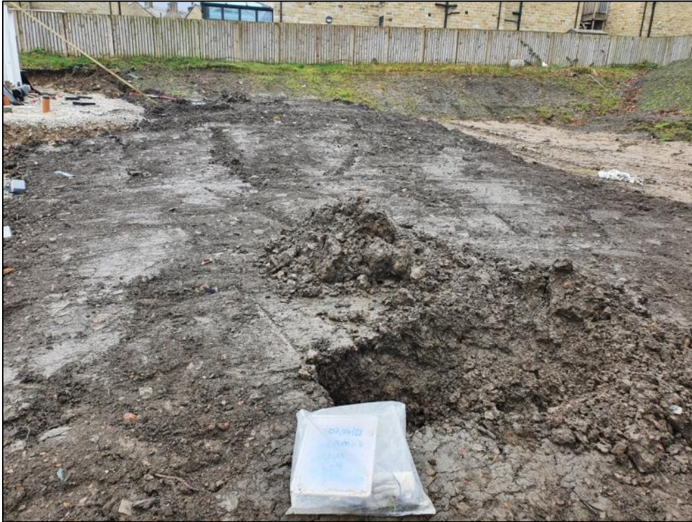
Plot 6 and 7: Wide view of validation trial pit.
