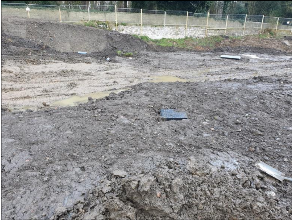
Plot 8 and 9: Wide view of validation trial pit location.
