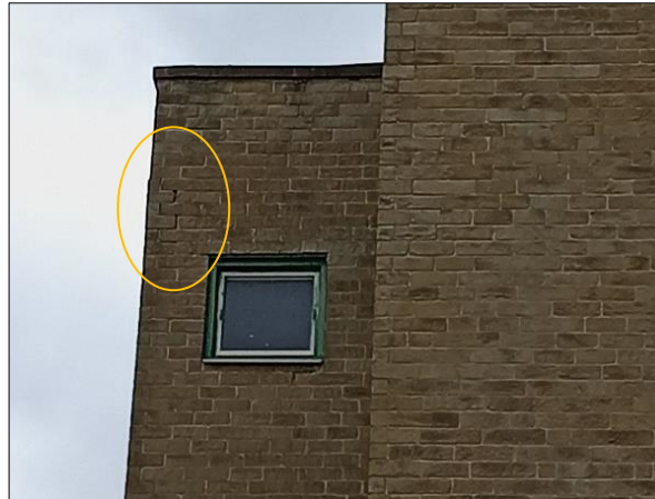
Figure 5 Gaps in mortar underneath windowsill to the south aspect.
