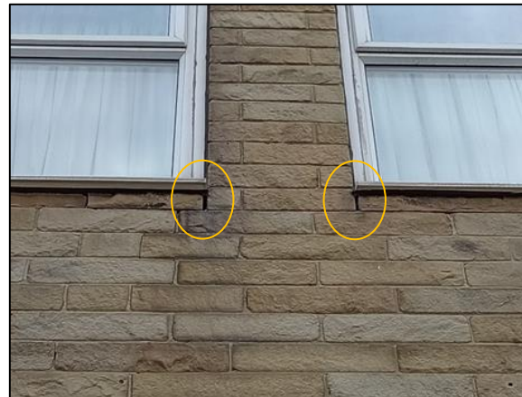
Figure 5 Gaps in mortar underneath windowsill to the south aspect.
