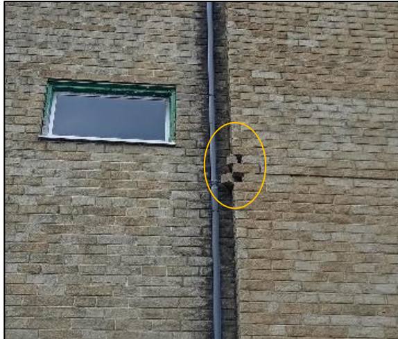
Figure 9 Dislodged bricks, corner to the west aspect.
