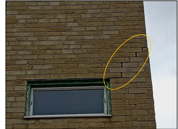
Figure 6 Gaps in mortar and above wooden fascia boards.
