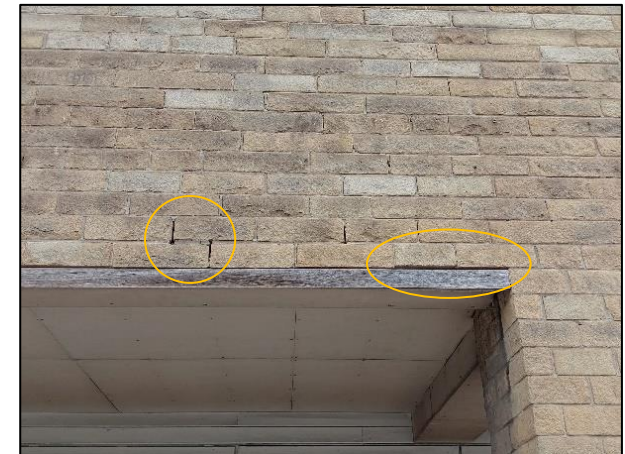
Figure 6 Gaps in mortar and above wooden fascia boards.
