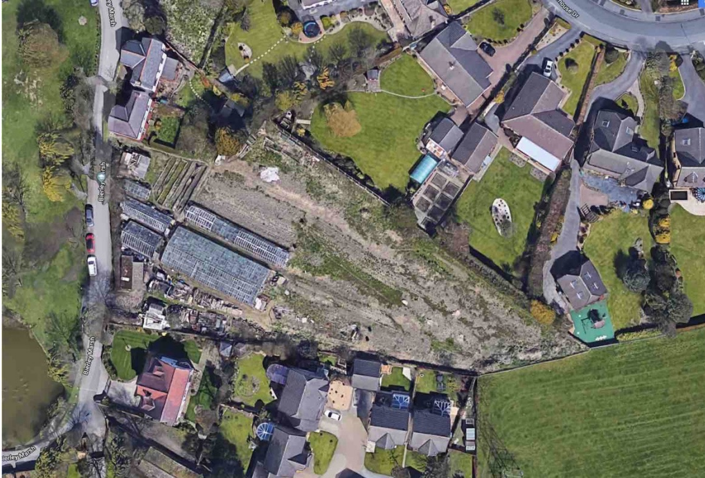
Aerial photograph illustrating the redundant nursery which has now been demolished.
