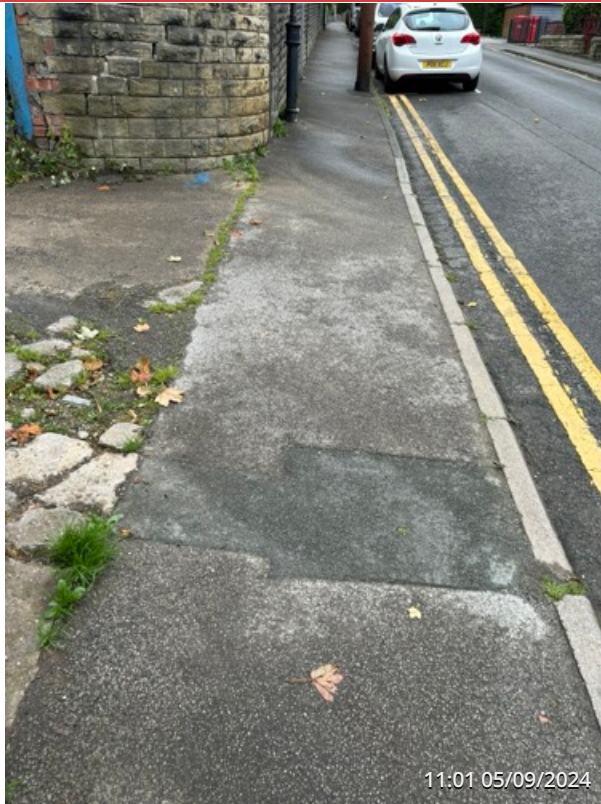
EXTERNAL SITE ENTRANCE AREA
