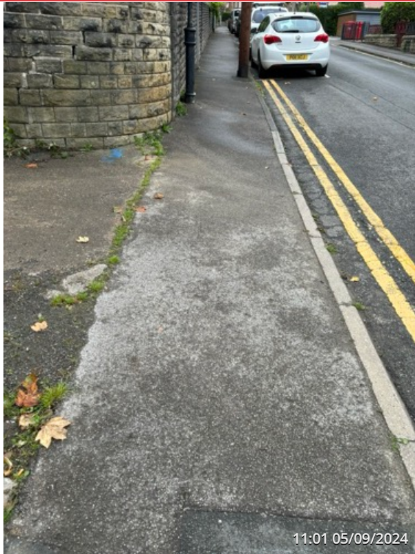
EXTERNAL SITE ENTRANCE AREA
