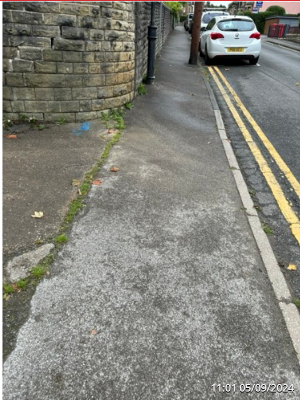
EXTERNAL SITE ENTRANCE AREA
