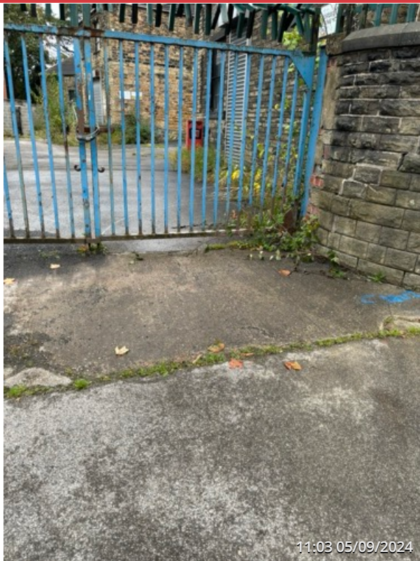
EXTERNAL SITE ENTRANCE AREA
