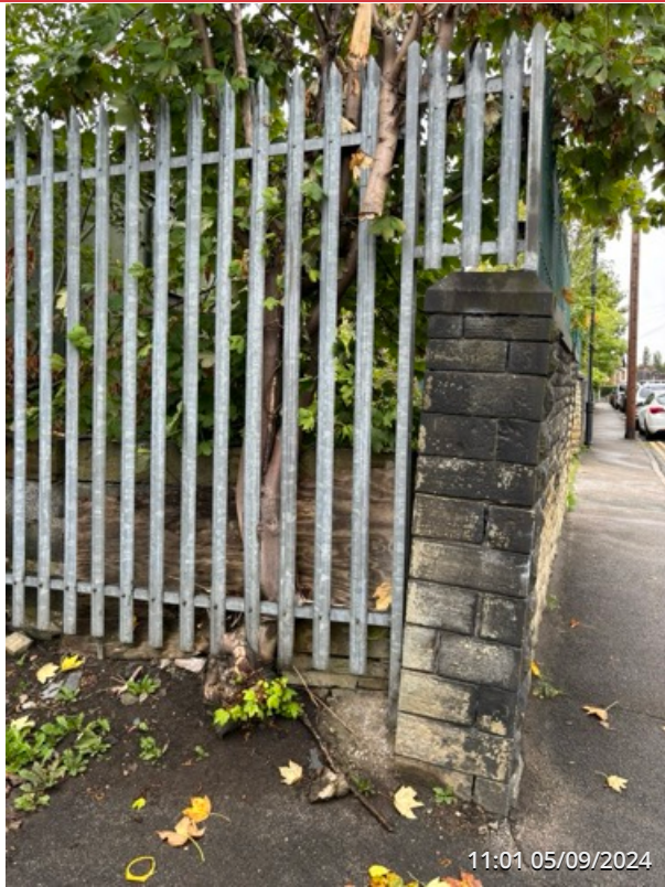
EXTERNAL SITE ENTRANCE AREA
