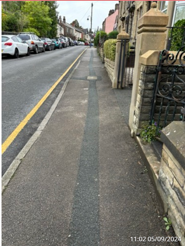
EXTERNAL SITE ENTRANCE AREA
