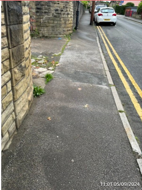
EXTERNAL SITE ENTRANCE AREA
