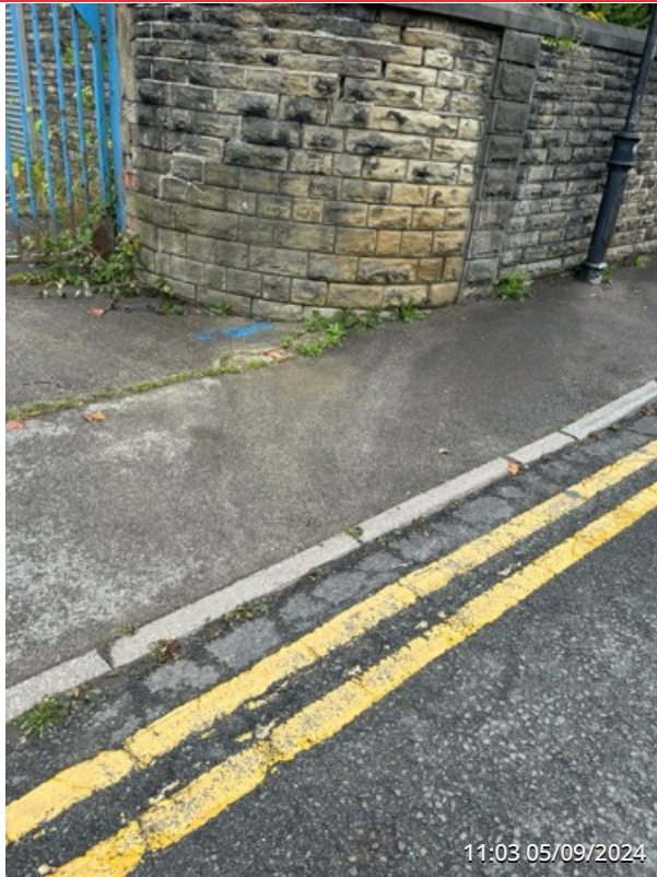
EXTERNAL SITE ENTRANCE AREA
