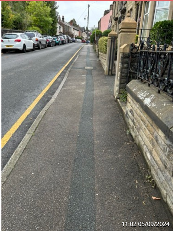
EXTERNAL SITE ENTRANCE AREA
