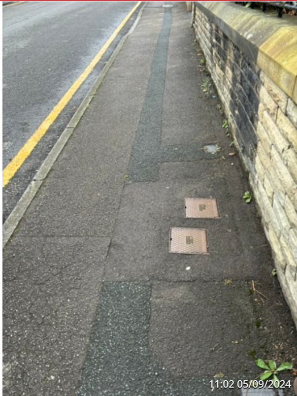
EXTERNAL SITE ENTRANCE AREA
