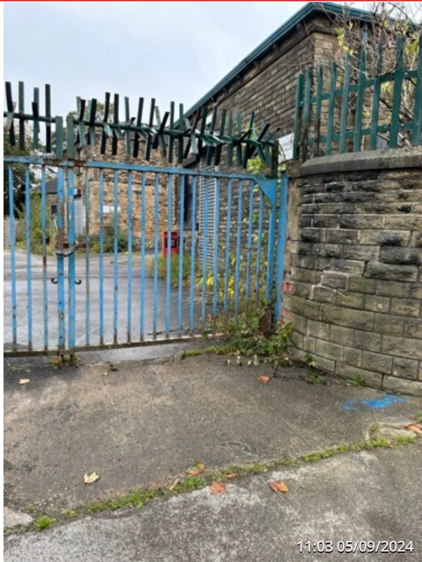
EXTERNAL SITE ENTRANCE AREA
