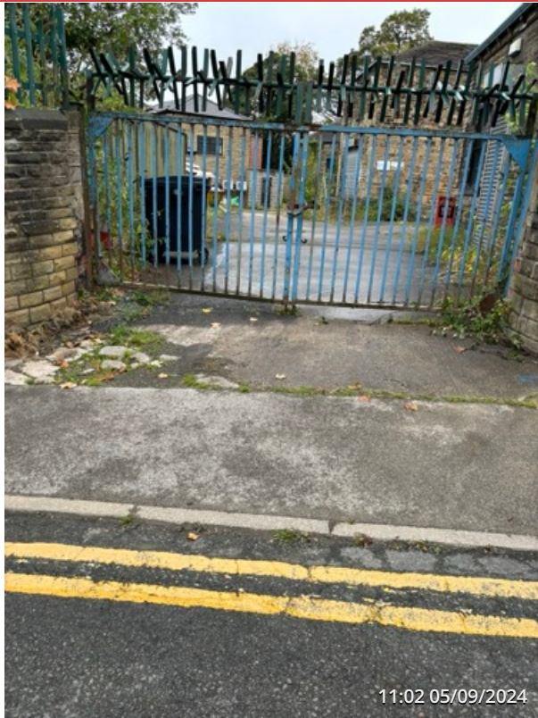
EXTERNAL SITE ENTRANCE AREA
