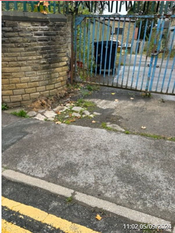
EXTERNAL SITE ENTRANCE AREA
