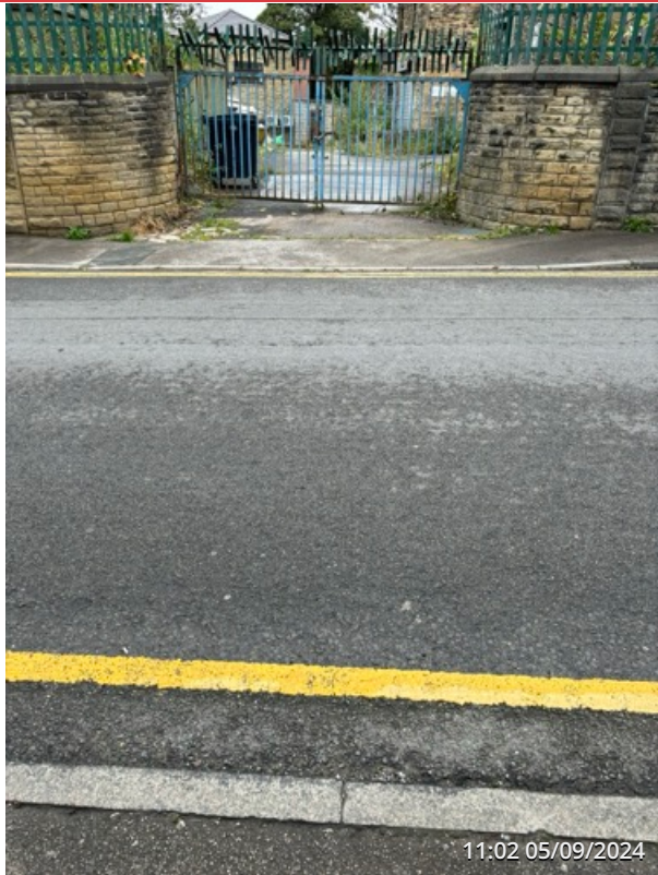
EXTERNAL SITE ENTRANCE AREA
