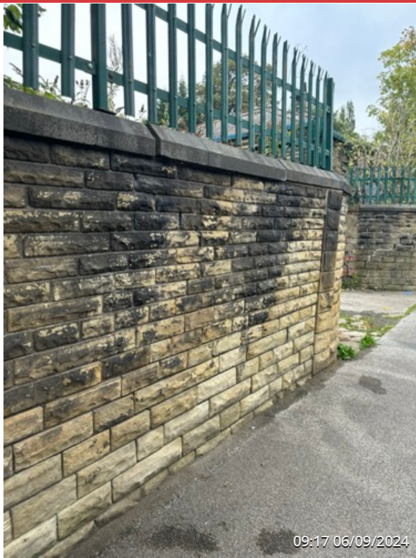
EXTERNAL SITE ENTRANCE AREA
