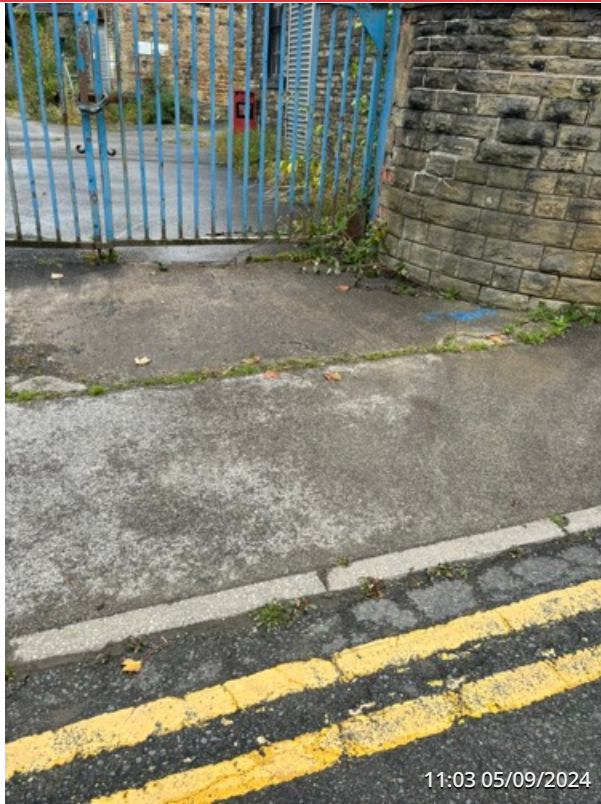
EXTERNAL SITE ENTRANCE AREA
