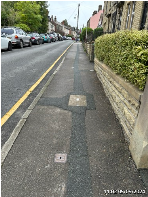
EXTERNAL SITE ENTRANCE AREA
