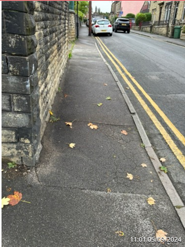
EXTERNAL SITE ENTRANCE AREA
