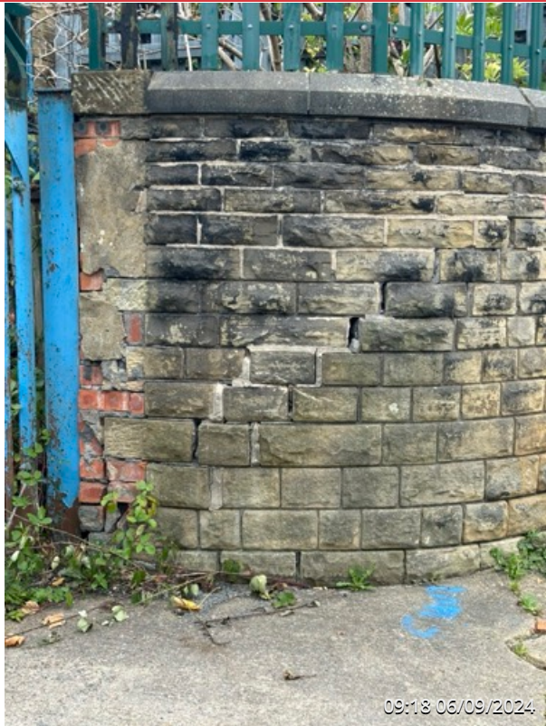
EXTERNAL SITE ENTRANCE AREA
