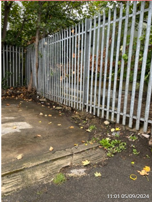
EXTERNAL SITE ENTRANCE AREA
