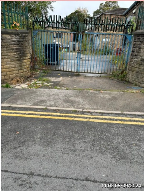
EXTERNAL SITE ENTRANCE AREA
