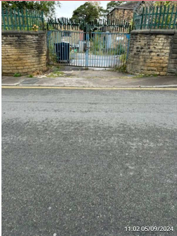
EXTERNAL SITE ENTRANCE AREA
