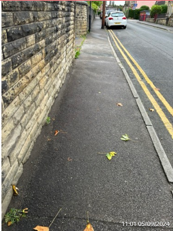
EXTERNAL SITE ENTRANCE AREA
