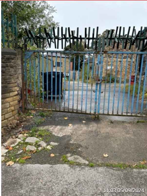
EXTERNAL SITE ENTRANCE AREA
