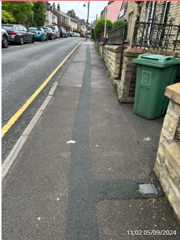
EXTERNAL SITE ENTRANCE AREA
