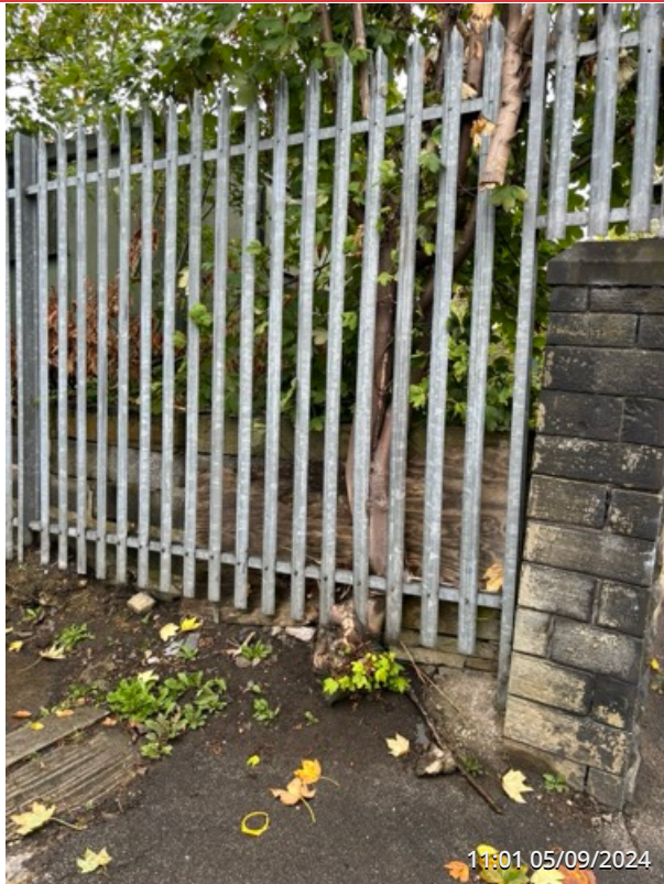
EXTERNAL SITE ENTRANCE AREA
