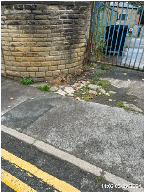
EXTERNAL SITE ENTRANCE AREA
