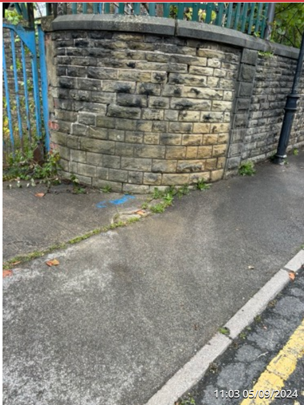
EXTERNAL SITE ENTRANCE AREA
