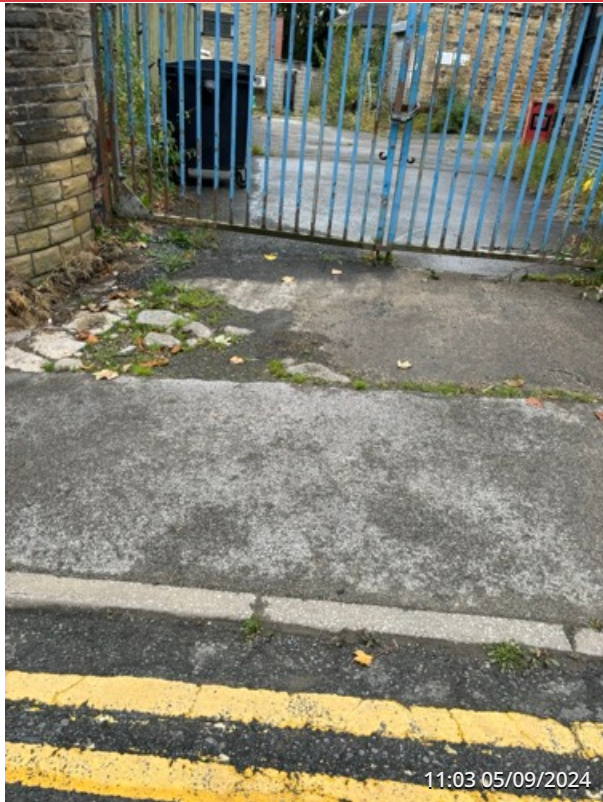
EXTERNAL SITE ENTRANCE AREA
