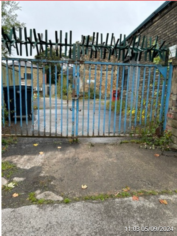
EXTERNAL SITE ENTRANCE AREA
