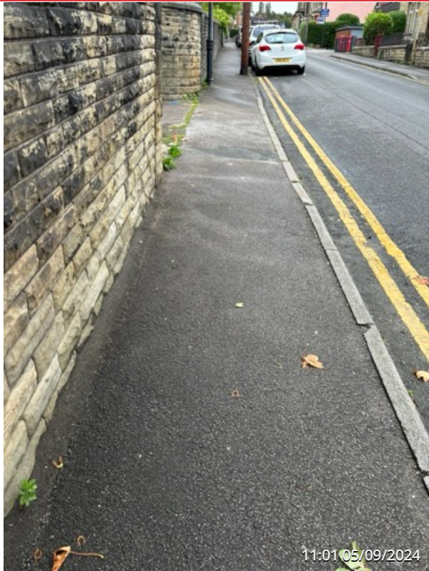
EXTERNAL SITE ENTRANCE AREA
