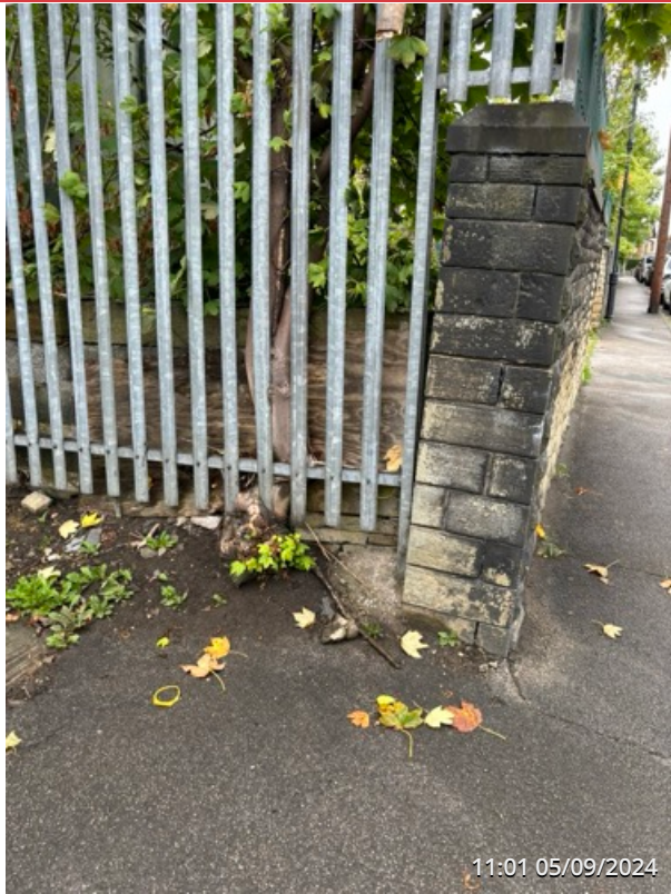
EXTERNAL SITE ENTRANCE AREA
