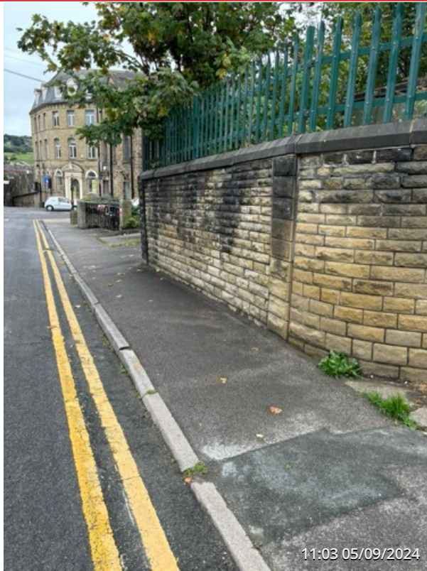
EXTERNAL SITE ENTRANCE AREA
