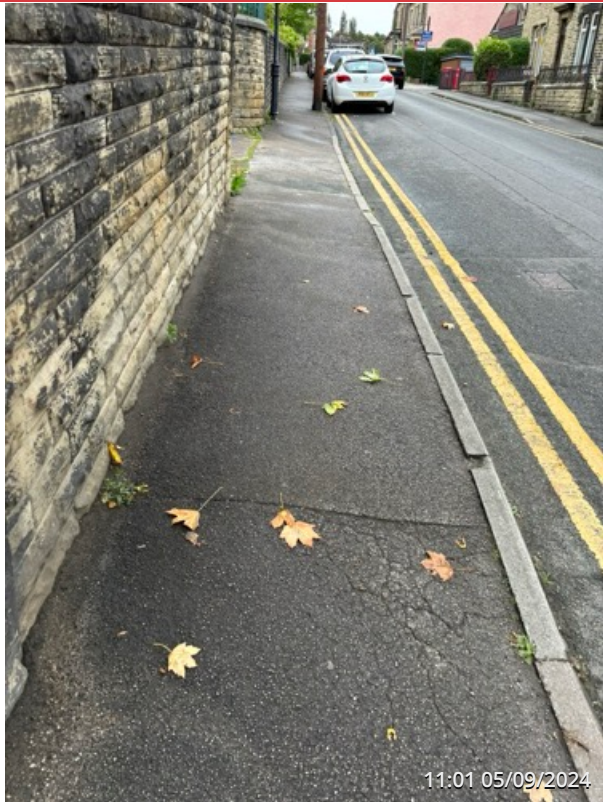
EXTERNAL SITE ENTRANCE AREA
