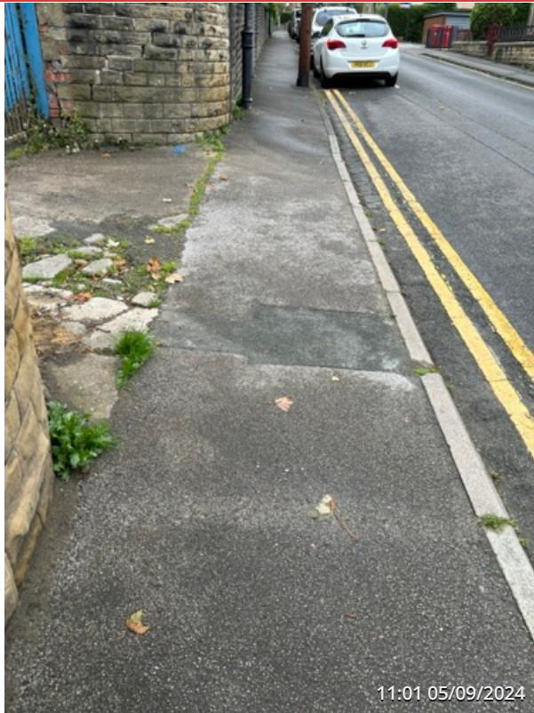
EXTERNAL SITE ENTRANCE AREA
