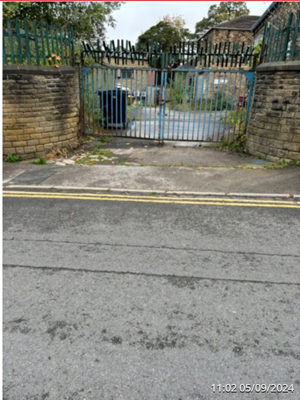
EXTERNAL SITE ENTRANCE AREA
