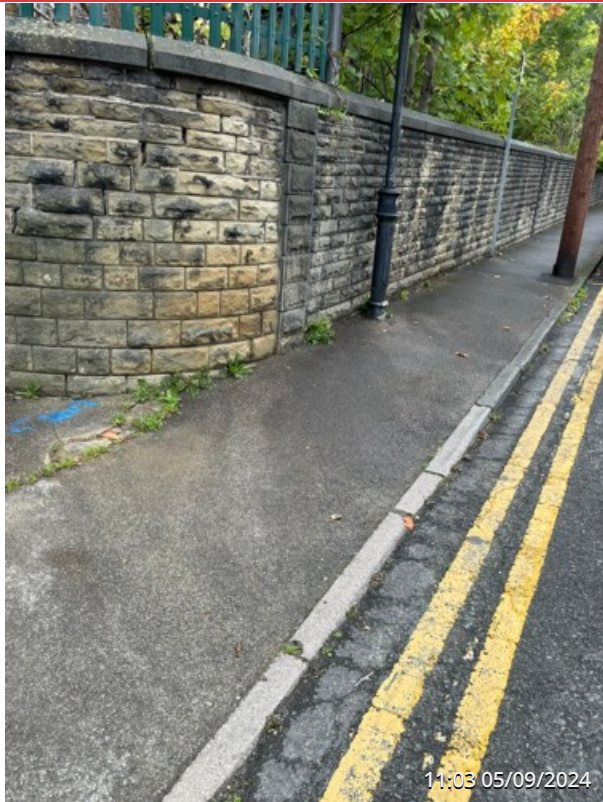
EXTERNAL SITE ENTRANCE AREA
