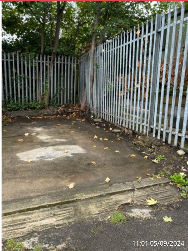
EXTERNAL SITE ENTRANCE AREA
