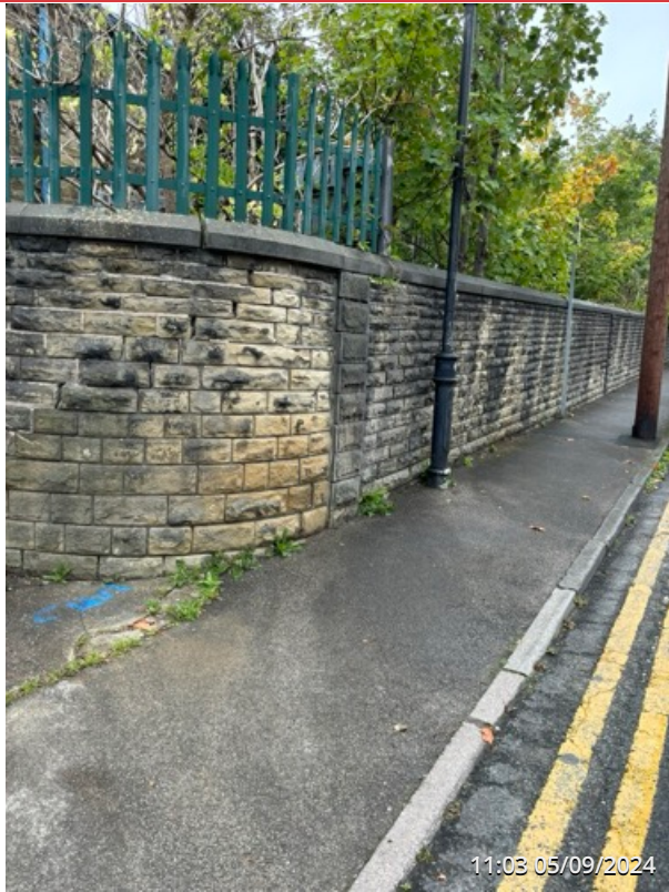
EXTERNAL SITE ENTRANCE AREA
