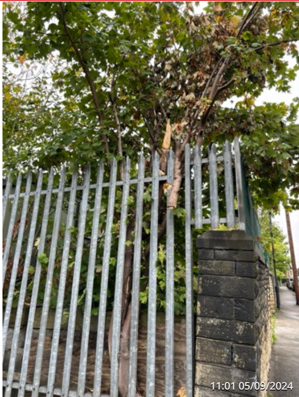
EXTERNAL SITE ENTRANCE AREA
