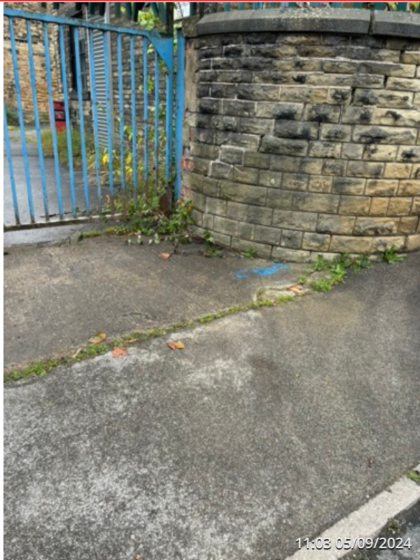
EXTERNAL SITE ENTRANCE AREA
