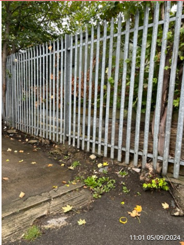
EXTERNAL SITE ENTRANCE AREA
