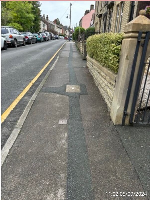
EXTERNAL SITE ENTRANCE AREA
