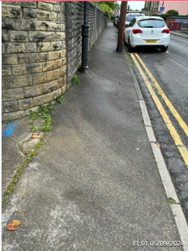
EXTERNAL SITE ENTRANCE AREA
