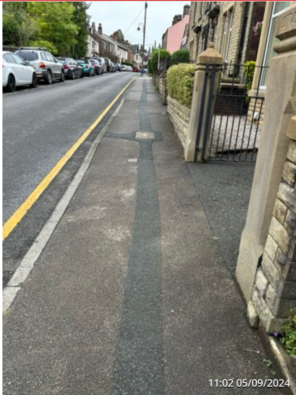
EXTERNAL SITE ENTRANCE AREA
