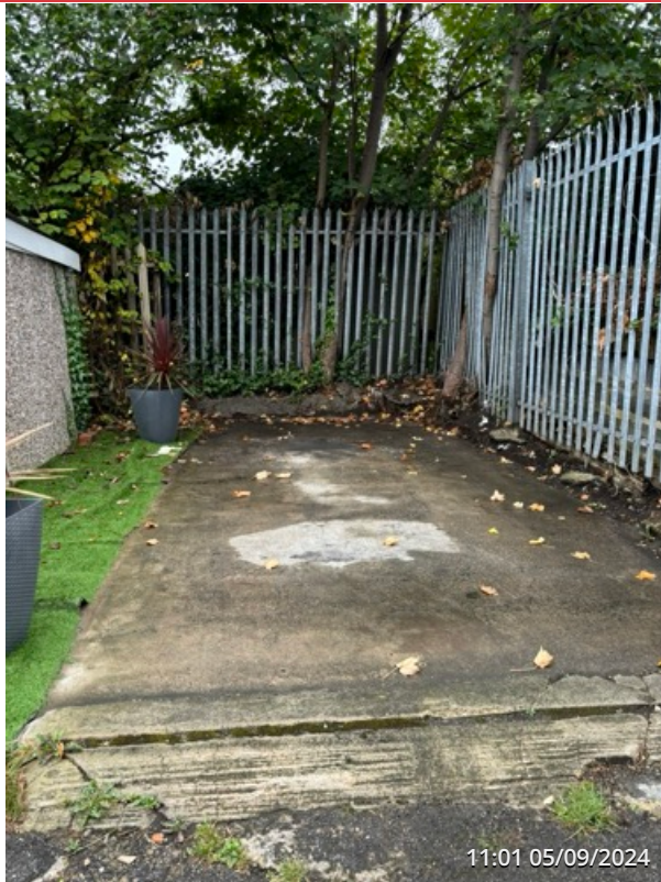
EXTERNAL SITE ENTRANCE AREA
