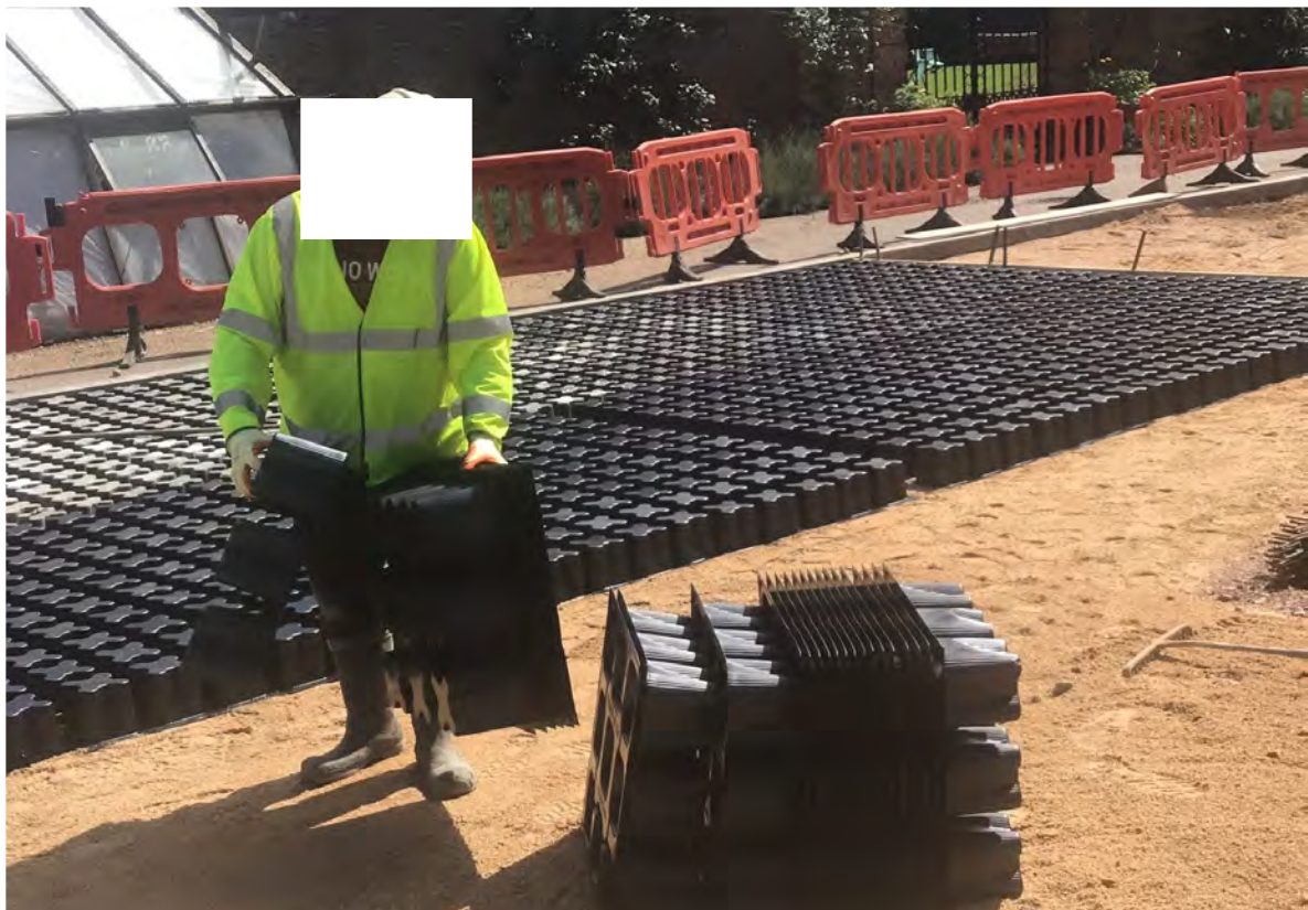
Fig. 12 Grasscrete GC2 void formers being removed from their nests, ready for installation
