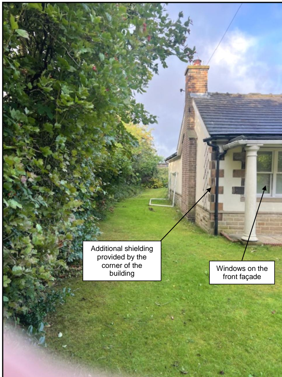
Photograph 4. Front façade of 79 Lathom Lane
