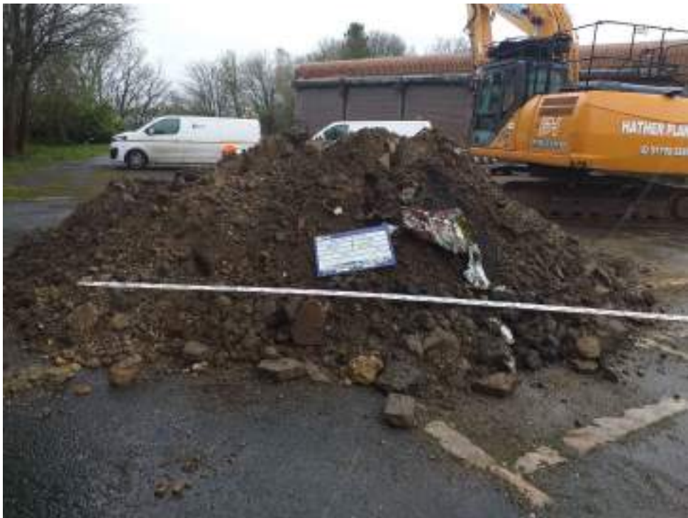
2: TP02 - looking into the pit and the arisings.
