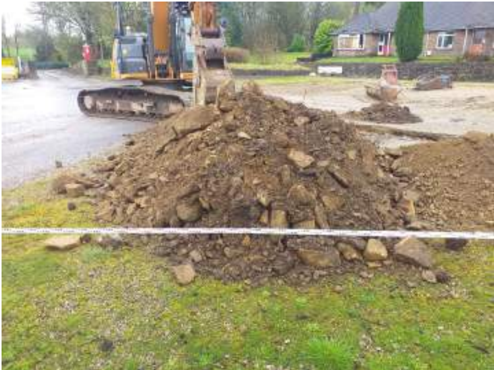
1: TP01 - looking into the pit and the arisings.
