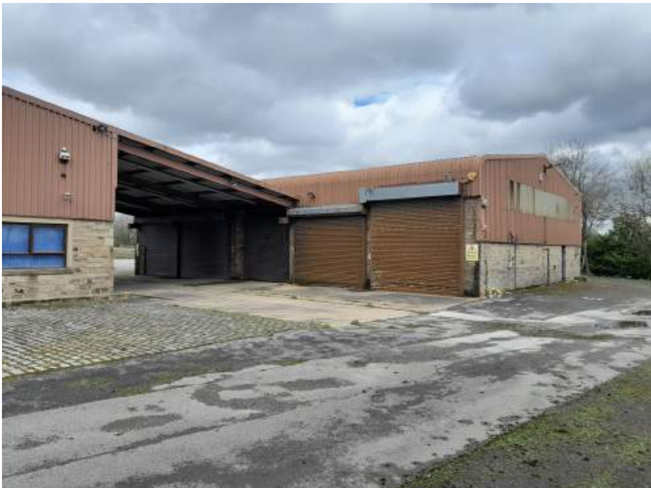
2: Looking southeast, towards the existing building onsite with the inspection pit inside.
