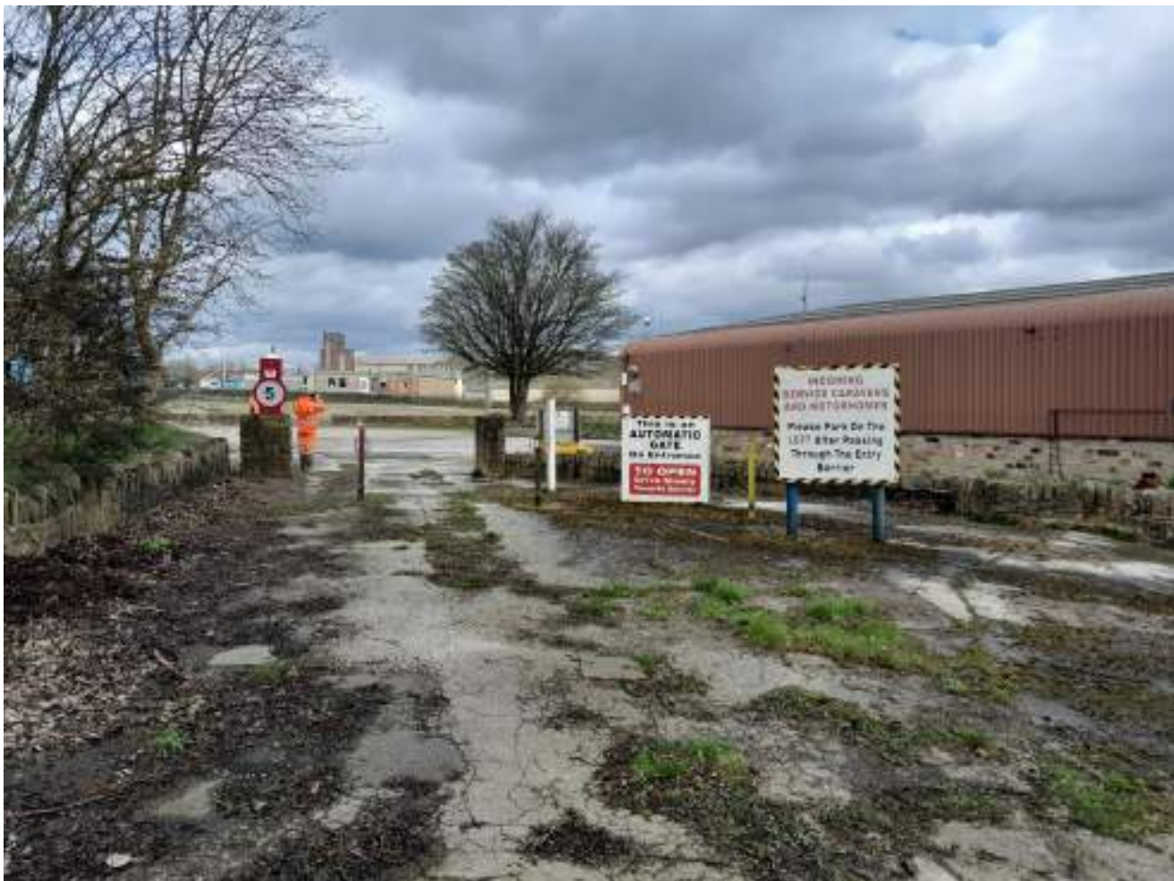
1: Looking north, onto the main access into the site.
