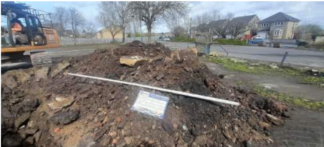
6: TP05 - looking into the pit and the arisings.
