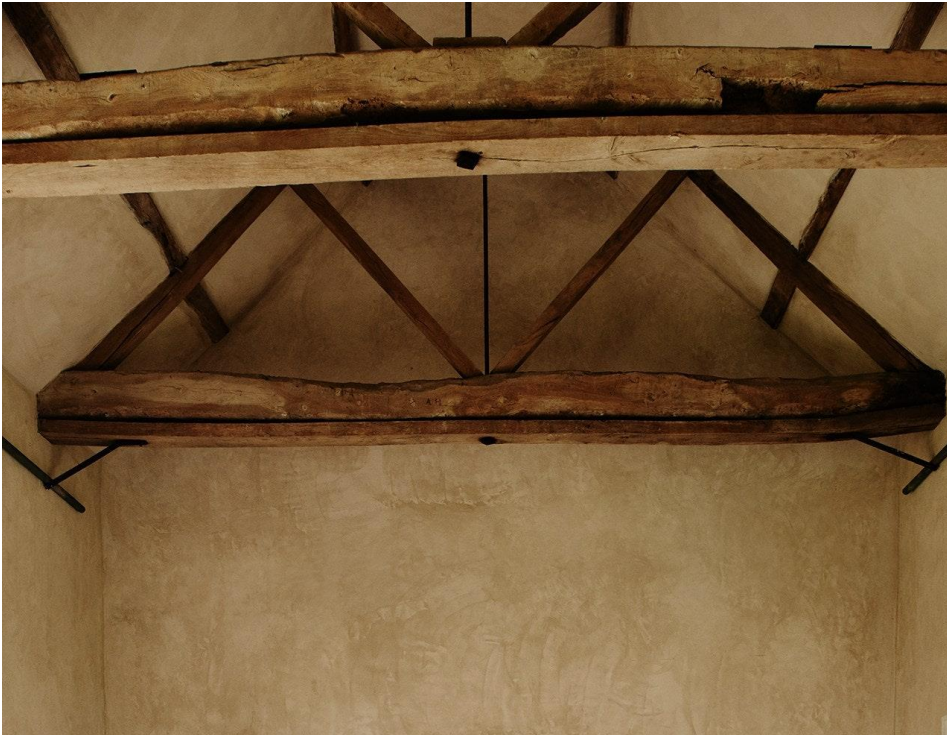
Photo 3: Example finish of a lime plastered wall with lime wash
