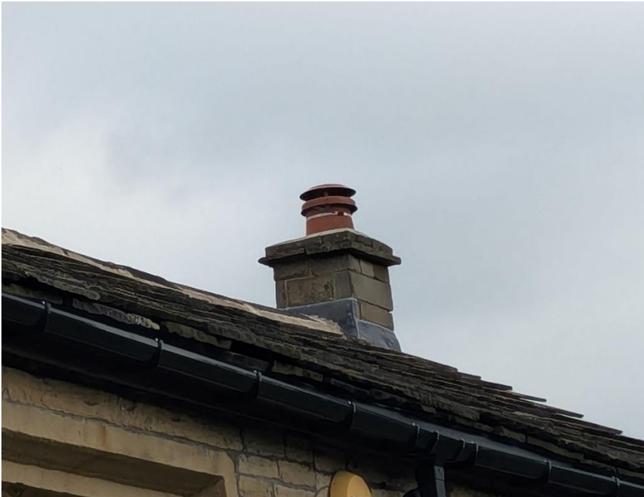
Photo 7: The other chimney of the property, disused and capped
