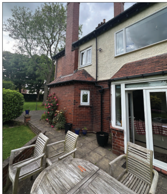
View to the side of the dwelling.
