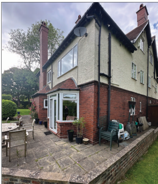
View to the side of the dwelling.
