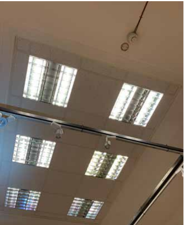
4.7.11 - Infilled rooflight opening to Gallery 1 (Rm. 87)
