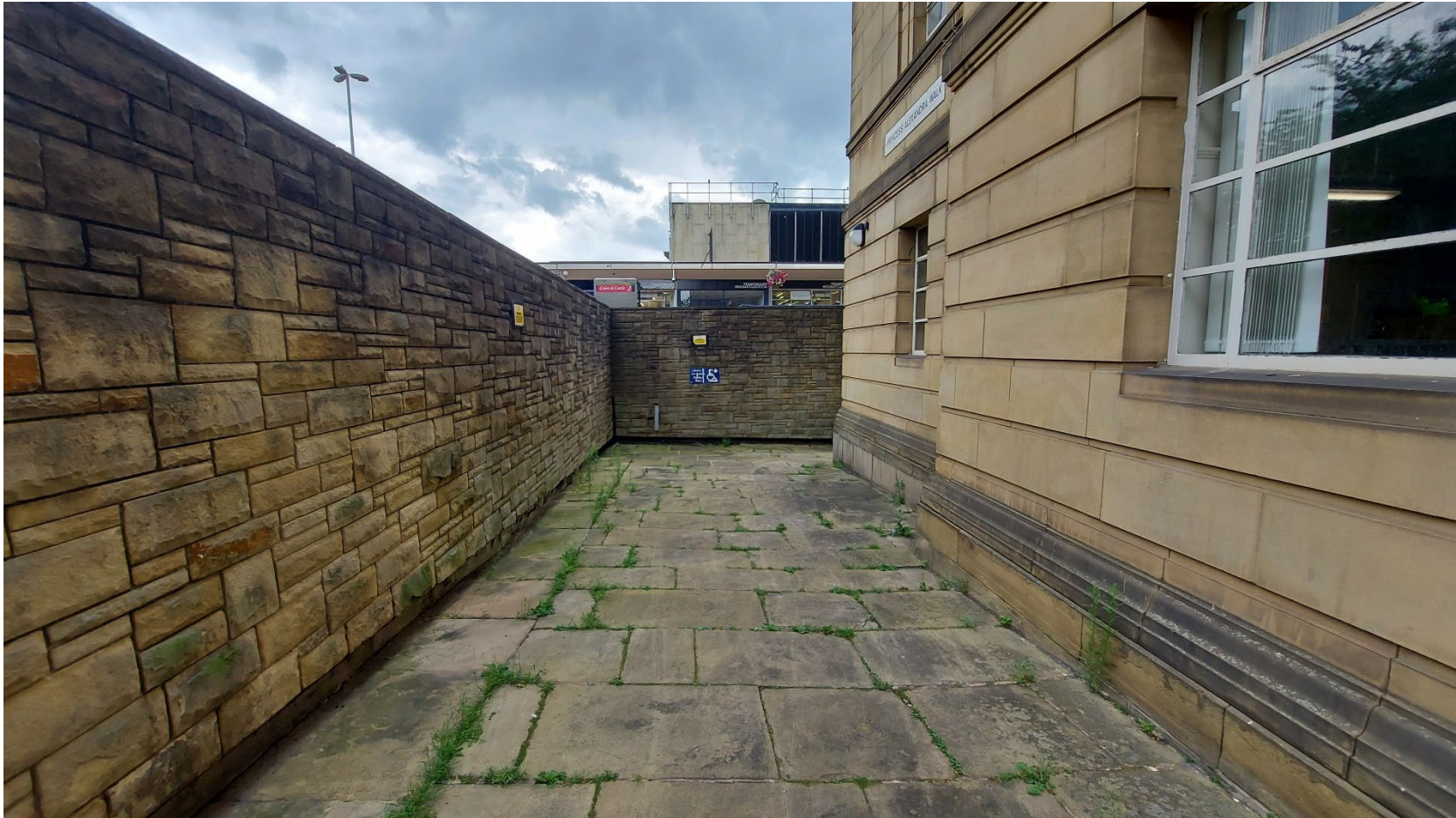
Plate 5: The area of the proposed outdoor classroom and modern retaining wall as existing.
