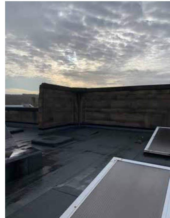
4.4.14 - Modern lanterns to roof
