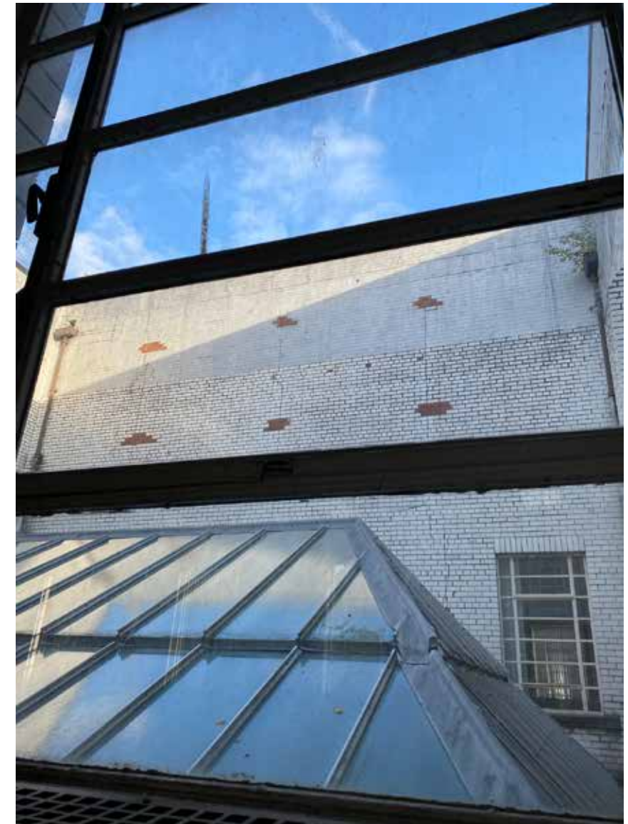
4.4.20 - Lightwell above atrium
