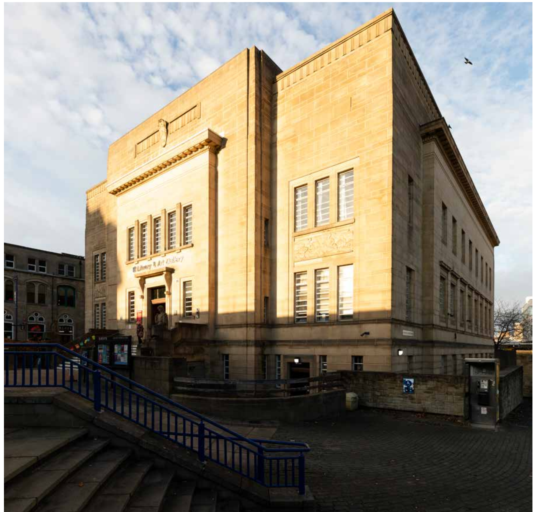
4.1.1.1 - Huddersfield Library and Art Gallery building
