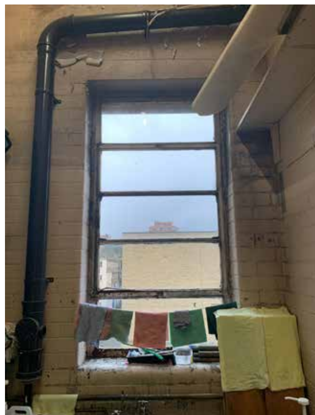
4.7.23 - Store / Service Room (Rm. 83)
