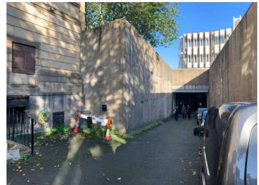
4.4.7 - Tunnel access below east elevation
