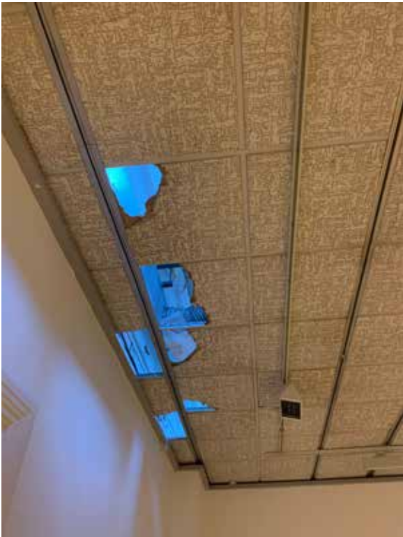
4.7.21 - Ceiling to Gallery 3 (Rm. 85)
