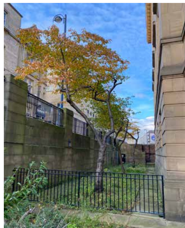
4.4.9 - West elevation and sunken garden
