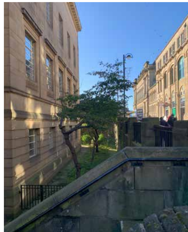
4.4.8 - West elevation and sunken garden
