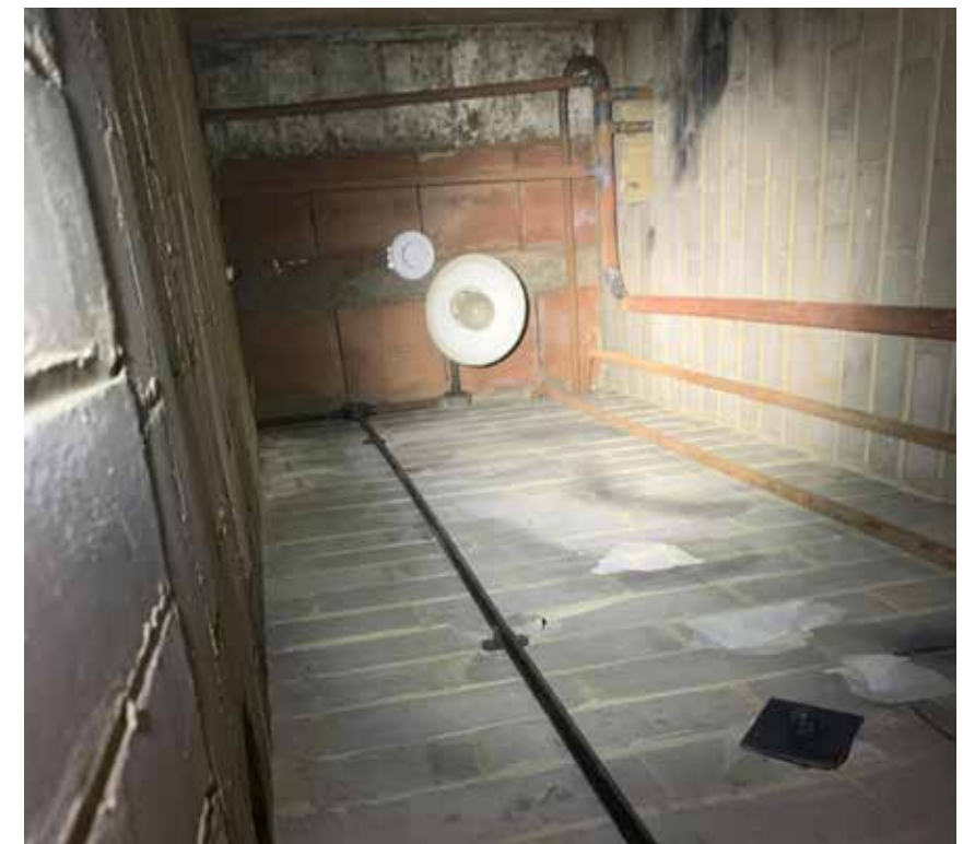
4.7.7 - Plant Space (Rm.89)
