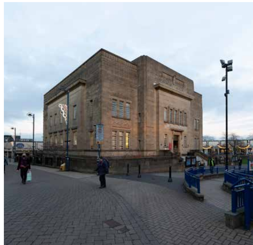
4.3.1 - Library and Art Gallery viewed from south-west
