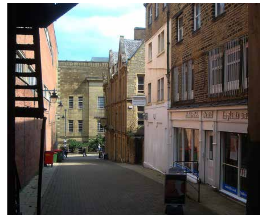
4.3.8 - View of west elevation from Albert Yard
