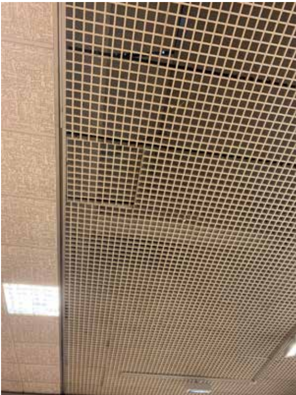
4.7.17 - Ceiling to Gallery 2 (Rm. 86)
