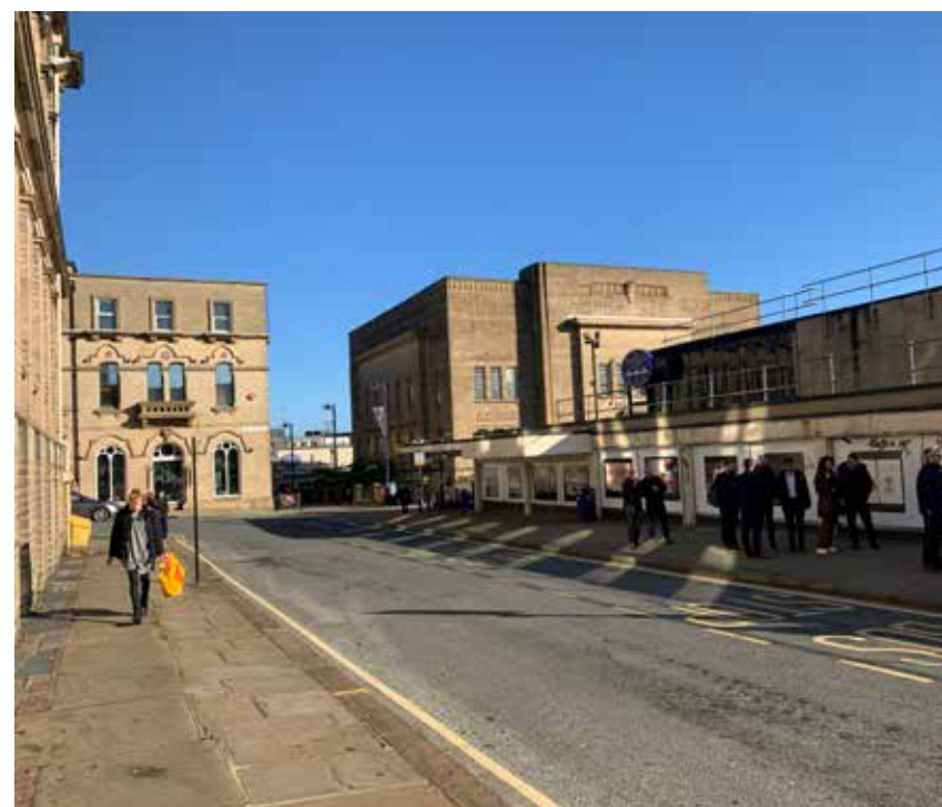
4.3.7 - View of building from Peel Street
