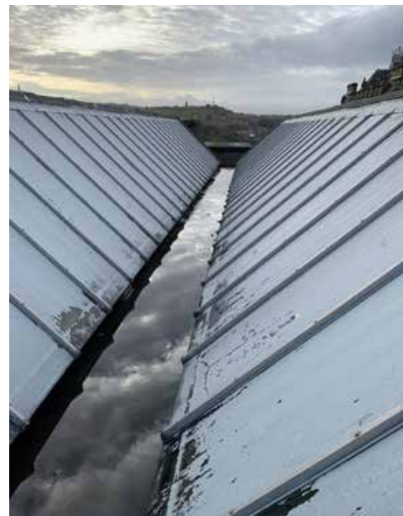
4.4.16 - Original lanterns to roof
