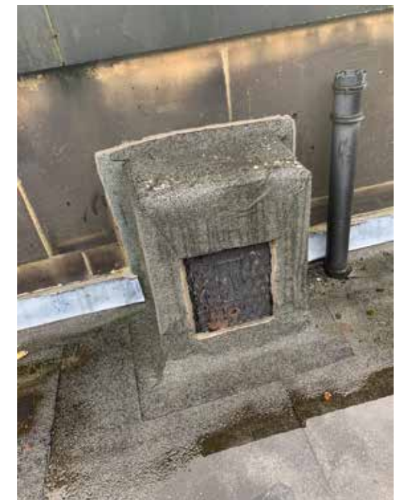
4.4.18 - Service access at roof
