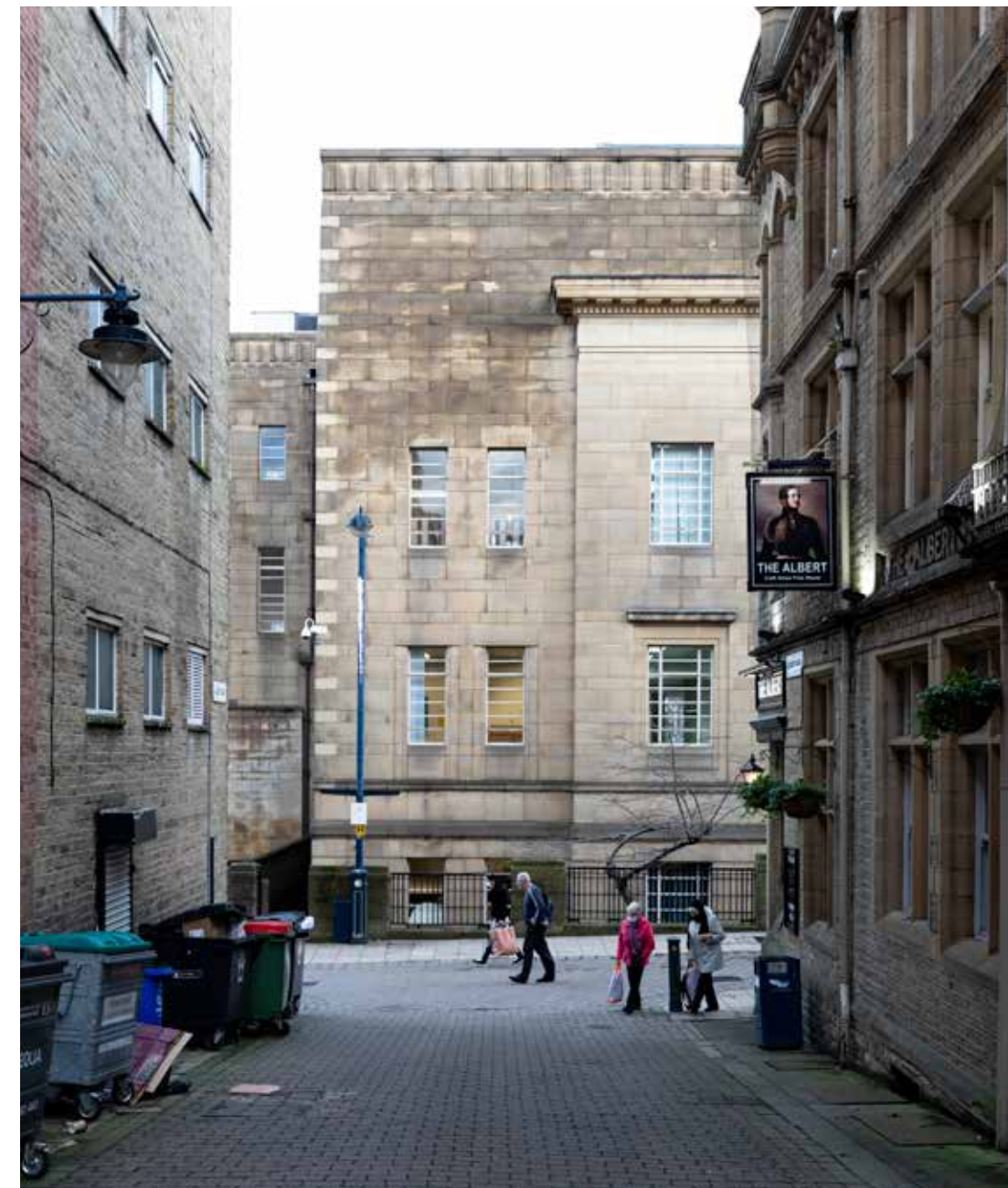
4.4.10 - East elevation from Albert Yard
