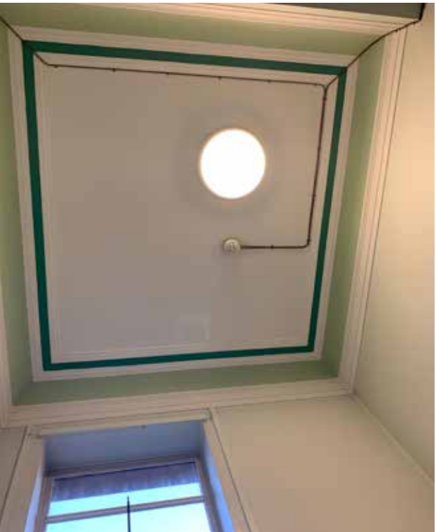
4.6.4 - Ceiling to First Floor Stair Lobby (Rm.71)
