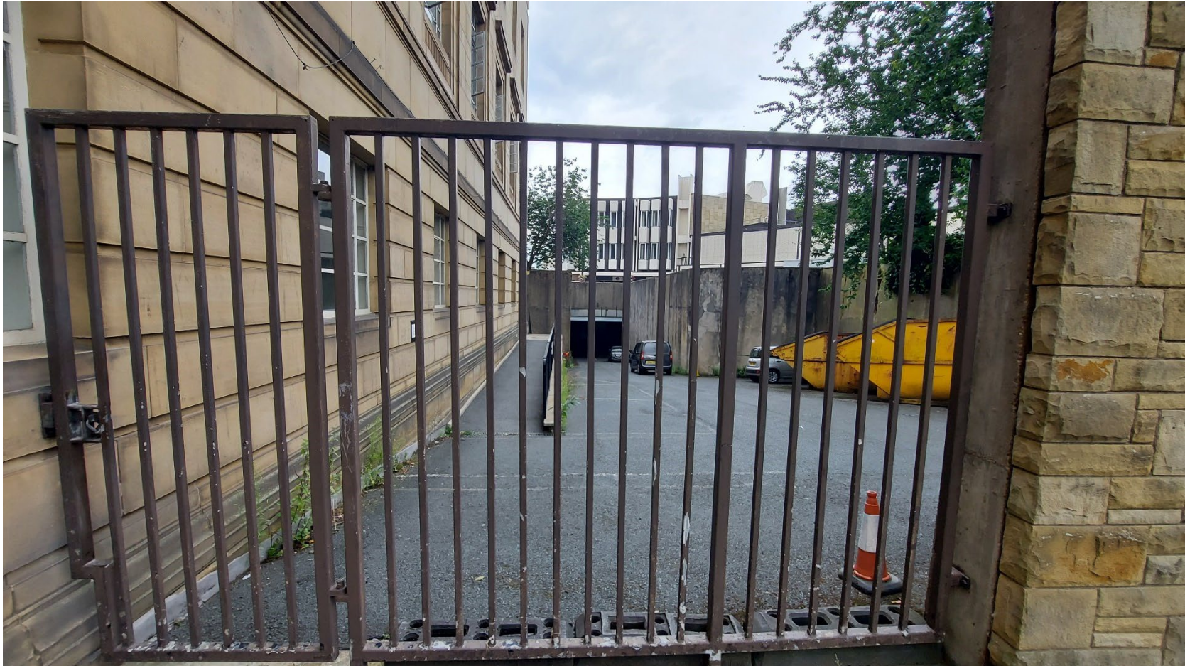
Plate 6: The area of the proposed outdoor classroom and modern retaining wall as existing.
