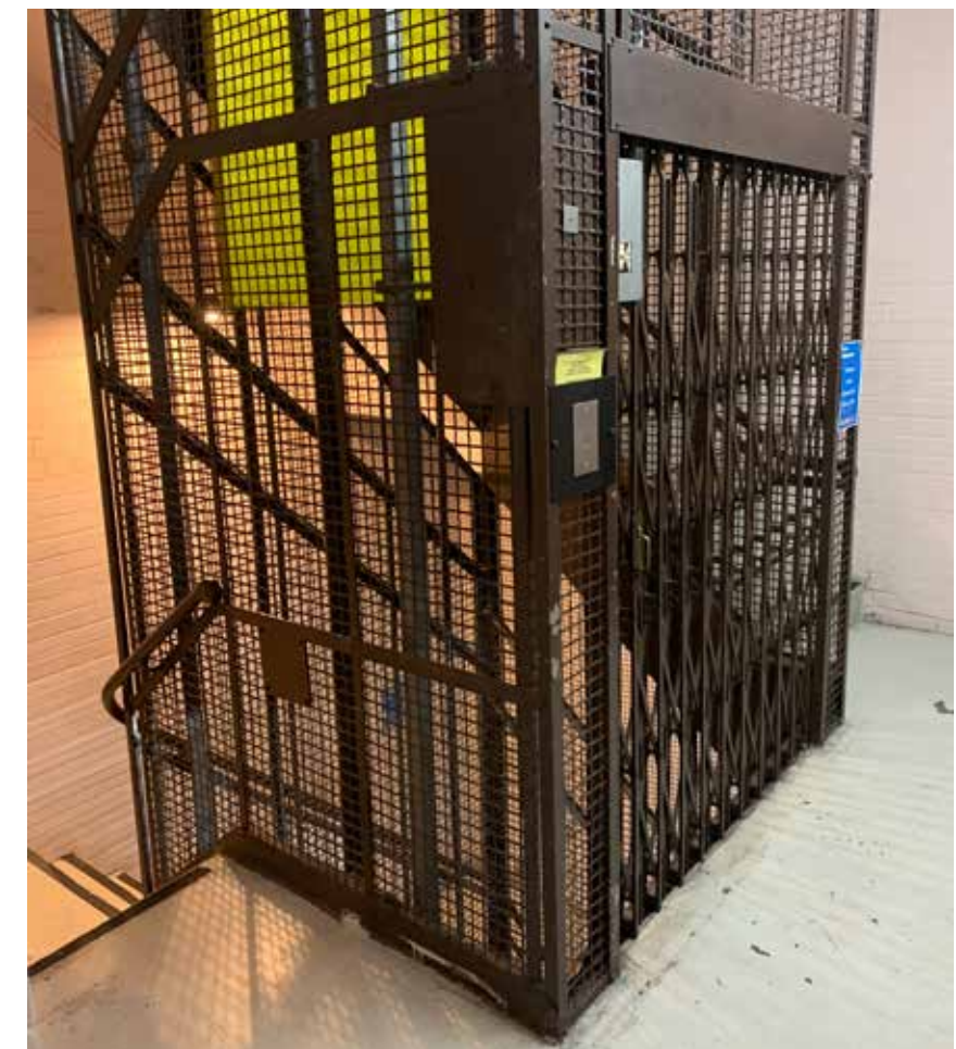
4.5.32 - Stair and Lift (Rm.40 & 41)
