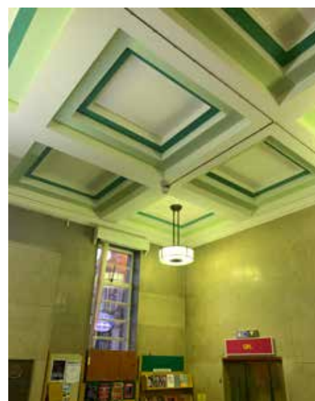
4.5.3 - Ceiling to Entrance Lobby / Reception (Rm.52)
