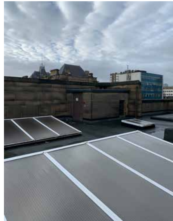
4.4.13 - Modern lanterns to roof
