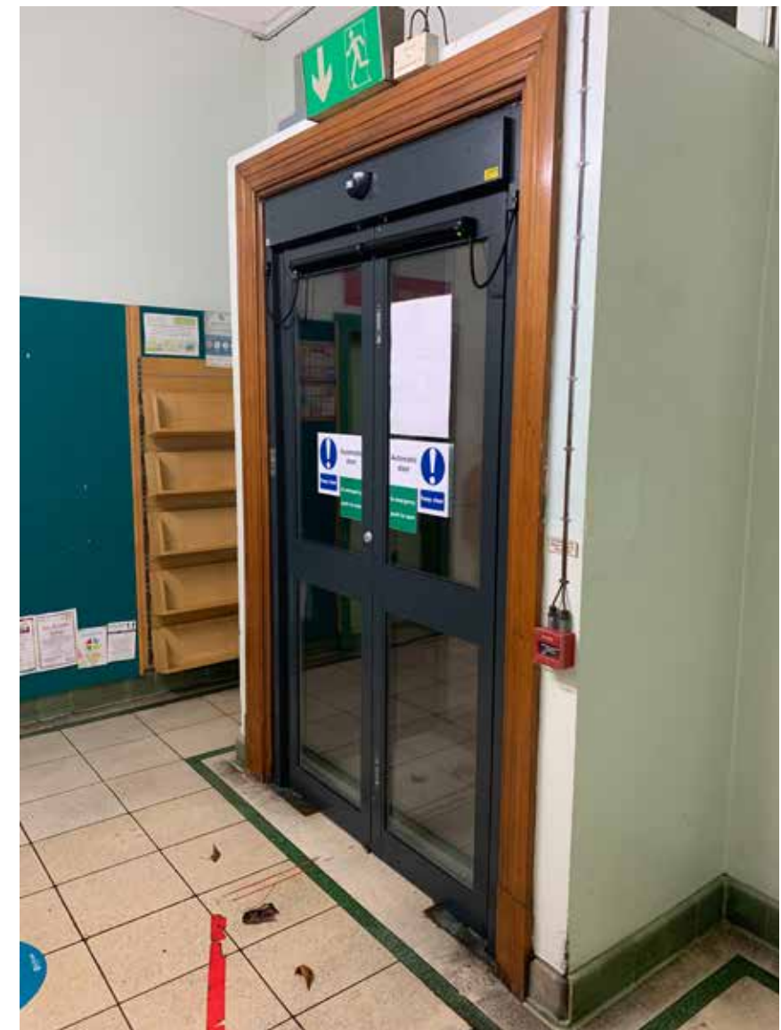
4.8.3 - East Entrance Lobby (Rm.28)
