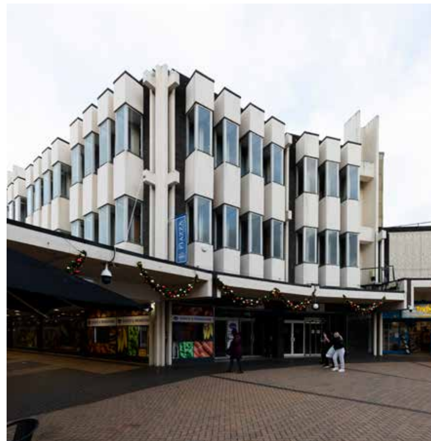
4.3.5 - Piazza Shopping Centre facing building's north aspect
