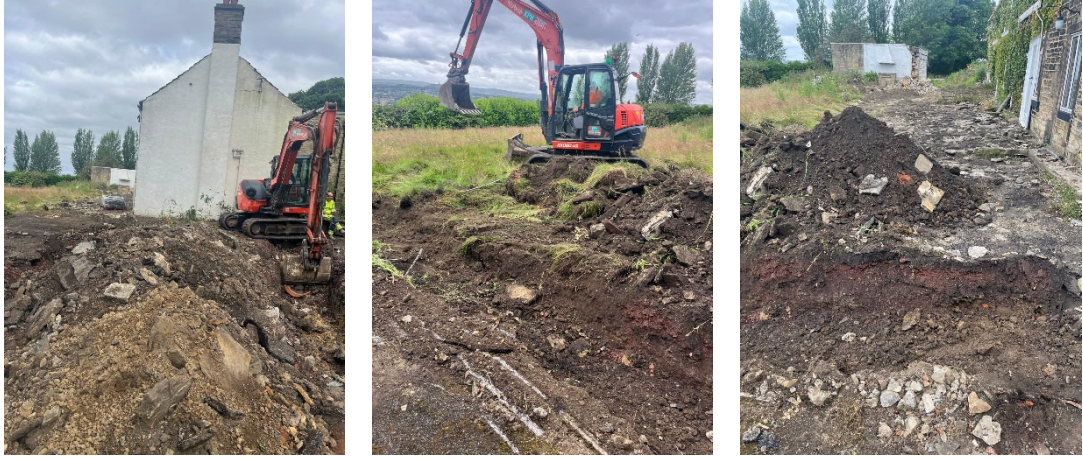
Figure 2: Photographs showing the start on site for the Permitted Development extensions
