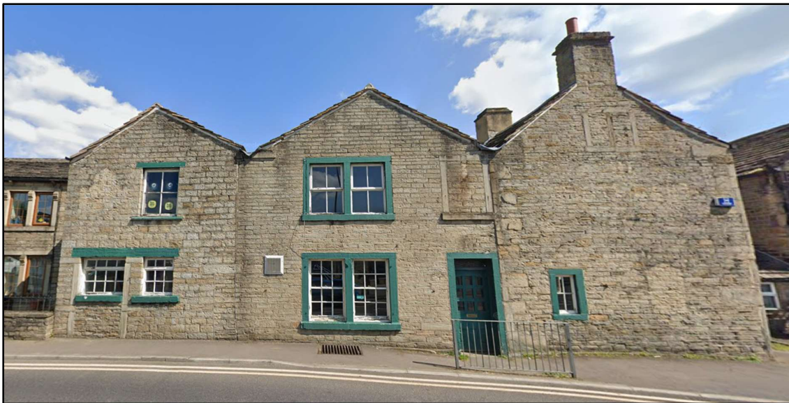
Figure 2 - Photograph of site from Huddersfield Road
