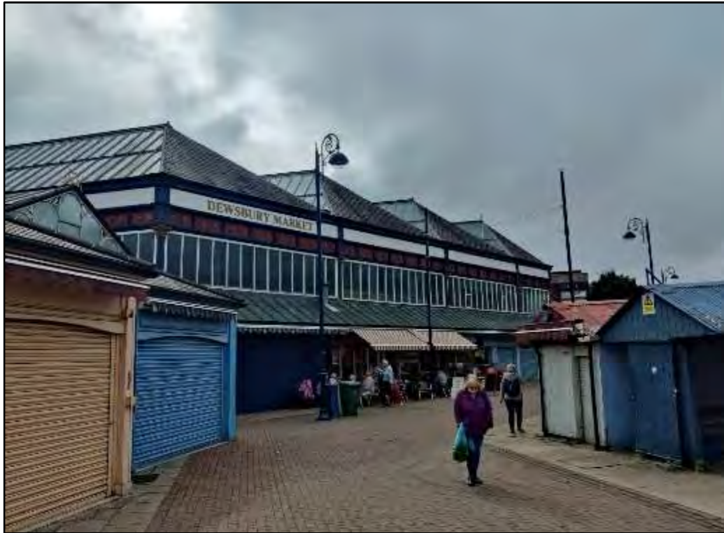
Photo G: View of the large indoor market building, facing south-east.
