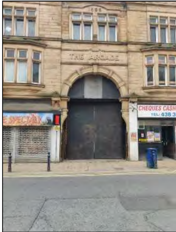
Photo I: View of the closed off Arcade area, facing south.
