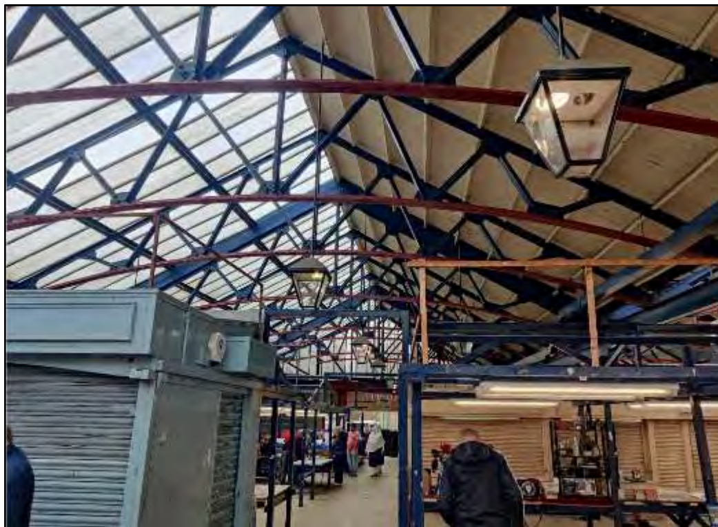
Photo F: View inside the large indoor market building facing north-east.
